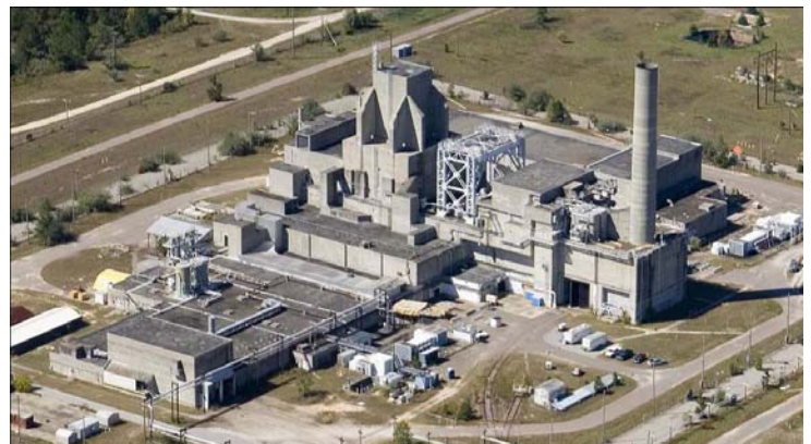
Typical nuclear reactor complex at SRS.
