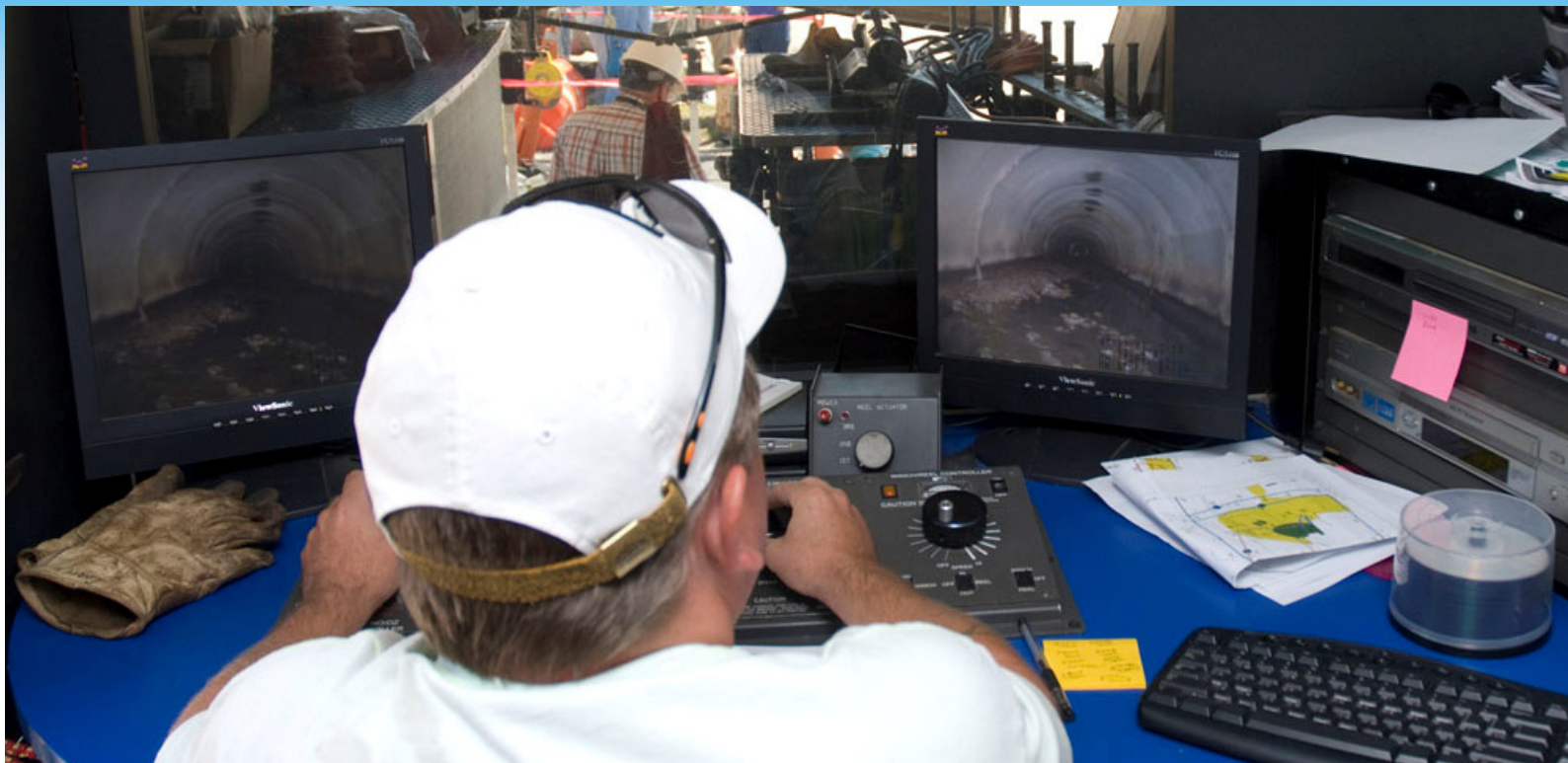
A worker views video footage of storm sewers from cameras set up by cleanup crews to evaluate current conditions before excavating soil and replacing piping.
