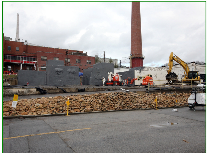
Phase One demolition work on Building 3026 being completed in December 2009. It left only the concrete hot-cell structures standing; they are scheduled to be removed in the next phase of operations.
