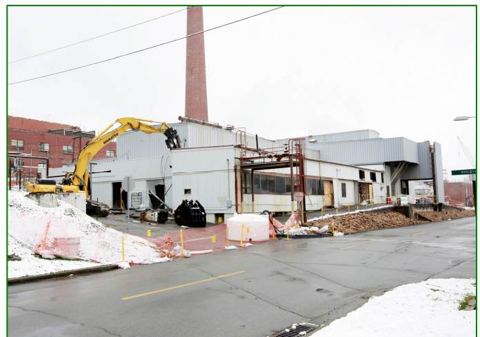
Pre-demolition activity taking place last year at Oak Ridge National Laboratory's Building 3026.
