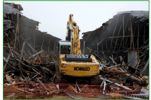
Building 9375 was demolished on February 8. To minimize particulate and dust, workers sprayed the work site with water.
