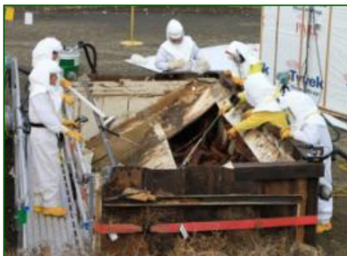
Box 82, one of two fiberglass-reinforced wooden boxes of radioactive waste that CH2M HILL is preparing for repackaging and removal from an underground storage trench.
