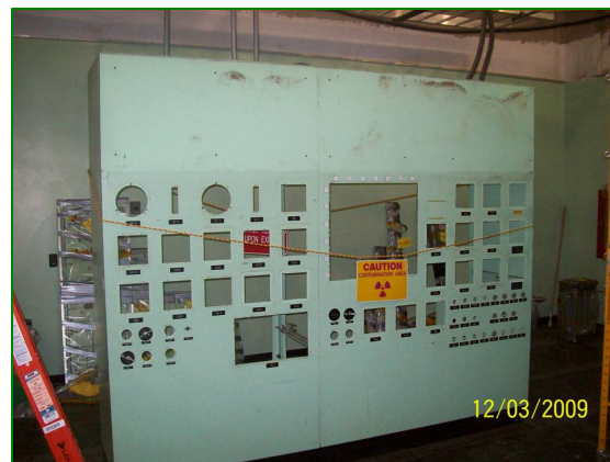
The partially removed control panel is pictured above. The work was completed in early January 2010.
