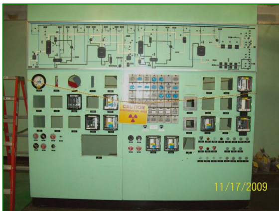
A free-standing control panel in the Main Plant Control Room identified for removal.
