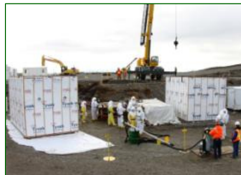
Waste retrieval in progress. The large boxes were fabricated to cover the deteriorated boxes of waste from adverse weather while the boxes and their contents are prepared for removal from the trench.
