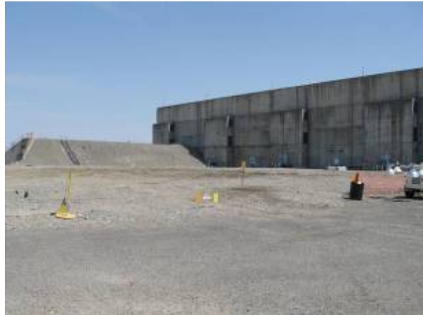
After demolition: Contractor CH2M HILL finished demolishing all 15 large tanks in July and disposed of the demolition debris in the Environmental Restoration Disposal Facility at the Hanford Site.
