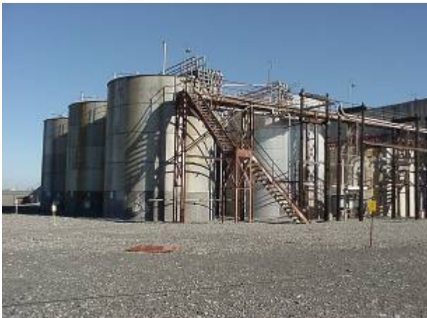
Before demolition: ten 100,000-gallon tanks and five 40,000-gallon tanks stood next to U Canyon, a former chemical separations plant at the Hanford Site in Washington State.
