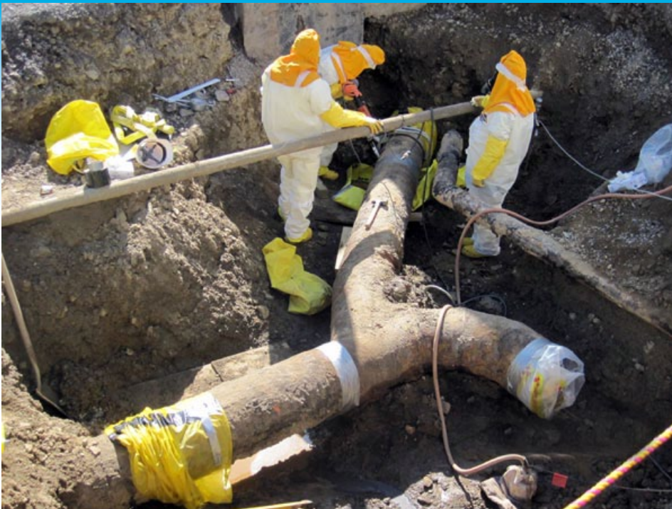
Workers excavate and remove a ventilation header that exhausts tank ventilation to the existing ventilation system. It will be replaced with new stainless steel piping.
