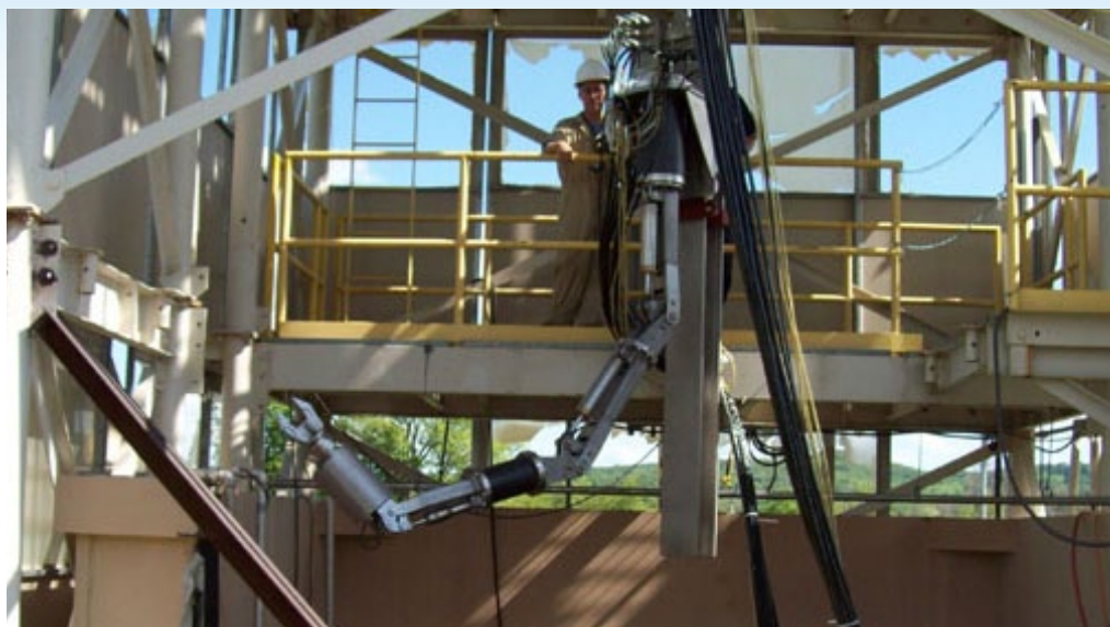
A worker oversees pre-deployment testing for the robotic arm at West Valley Demonstration Project.
