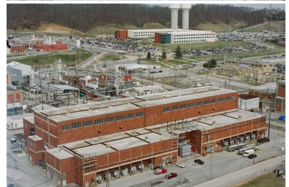
Top photo: Oak Ridge National Laboratory's central campus has been a priority for Recovery Act-funded cleanup.
