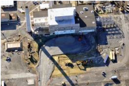
Removal of contaminated soil under the former location of the K East Reactor Basin This aerial shot (left) shows heavy equipment (right) excavating contaminated soil from a site next to the K East Reactor where a basin once stored 2,300 tons of spent nuclear fuel and radioactive sludge.
