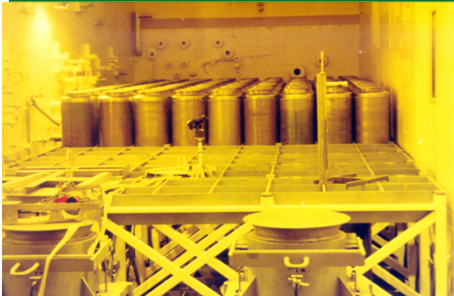
275 HLW Canisters in Safe Storage in Main Plant Process Building
