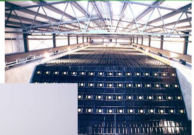
71-gallon drums of cemented waste in storage at the on-site "Drum Cell"
