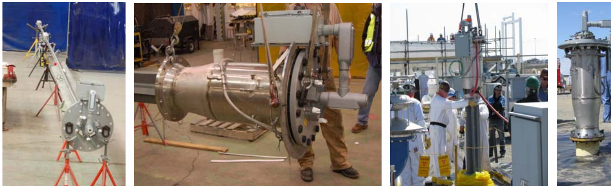
AN 102 Corrosion Probe Fabrication ⇒ Installation
