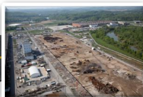
2010: Building K-25 West Wing demolished
