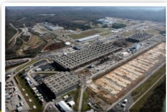
2011: Began Building K-25 East Wing demolition
