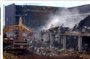
2006: Building K-29 at ETPP demolished
