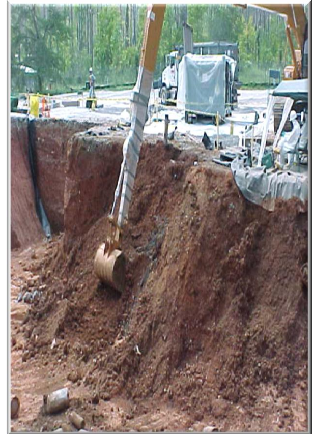
K-1070-B Burial Ground Excavation
