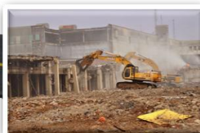
2008: Building K-25 West Wing demo begins
