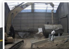
2012: Tank W-1A at ORNL removed
