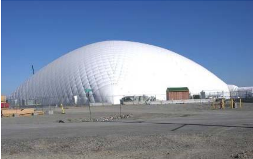
Weather Enclosure In Place November 5, 2007
