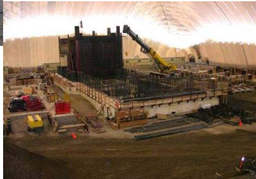
Shield Wall Formwork in Progress March 10, 2008
