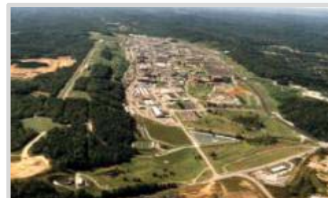
Y-12 National Security Complex
