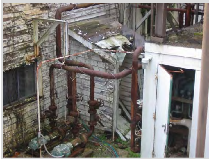
ORNL 3026 Wooden Superstructure
