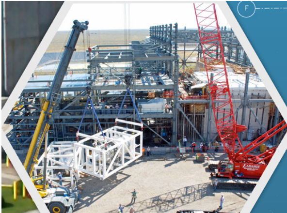
Construction of the Salt Waste Processing Facility at the Savannah River Site. Construction is planned for completion in 2015.
