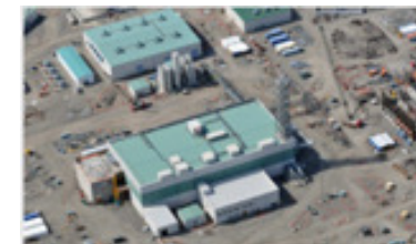
3. Low Activity Waste Vitrification Facility
