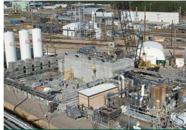
Construction of the Sodium Bearing Waste Treatment Facility at Idaho. SBWF construction is completed and operations initiated in April, 2012.
