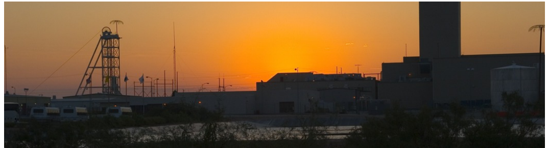
Surface facilities at WIPP near Carlsbad NM
