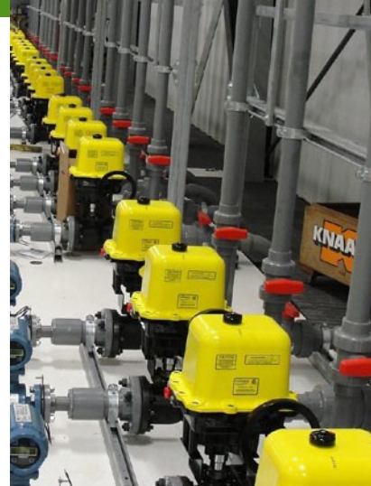
Equipment inside a groundwater treatment facility at Hanford.
