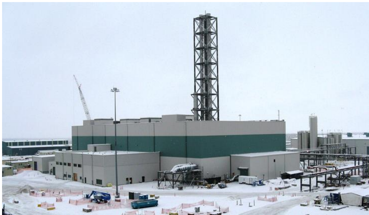
Figure 6-4. The Hanford LAW Facility under Construction in November 2010
