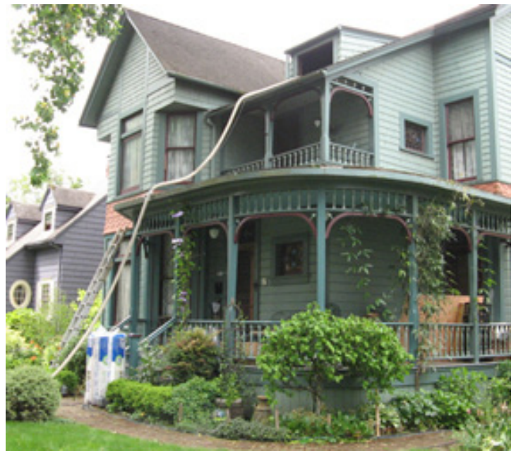
Insulation is blown into the home of Roy and Kim Fox in Portland, Ore. EcoTech modified its equipment to avoid damaging the home, which was built in 1884. | Photo courtesy of Roy Fox
