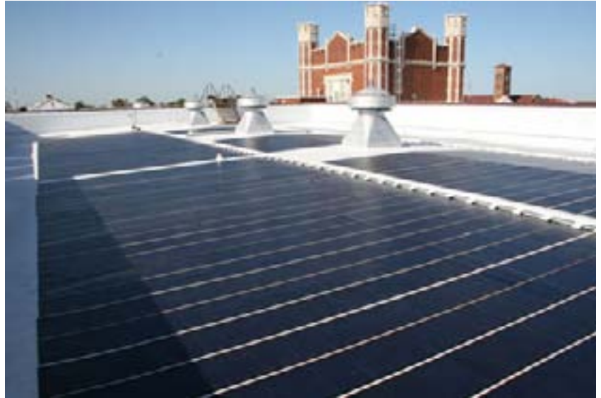
View of the solar panel system atop Warren Easton Senior High School in New Orleans
