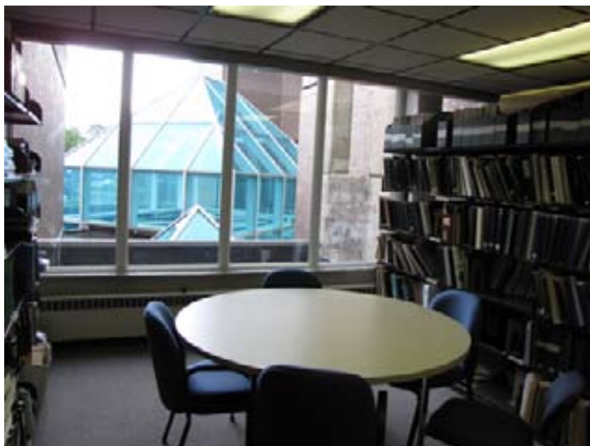
Low emissivity, double pane, fiberglass windows in Newark, Del.'s municipal building. I Photo courtesy of Carol Houck
