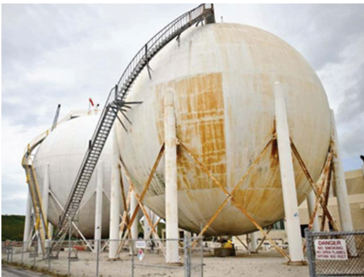
Through EECBG funding, the existing Miami-Dade County water treatment facility. | Photo courtesy of Miami-Dade County
