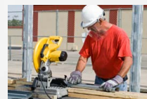
Power for tools for the work site
