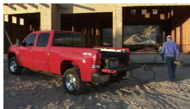
The onboard generator provides a work site with 15 kW of exportable power
