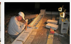
Emergency electricity and lighting
