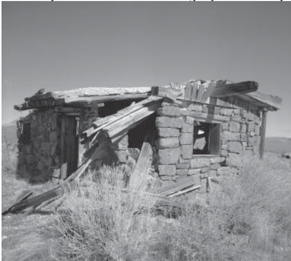
Ruins of herdsman's cabin at Tippihah Spring. Source: DOE, Nevada Operations Office.
