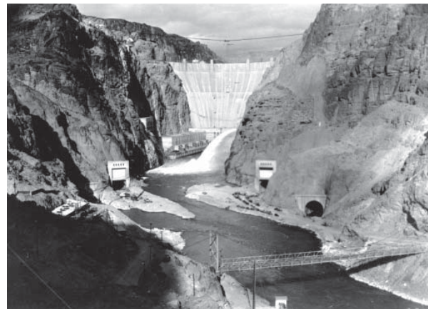
Hoover Dam. Source: Nevada Historical Society.
