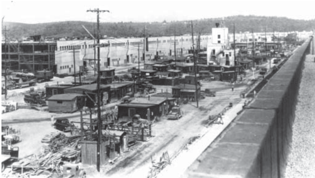
K-25 Gaseous Diffusion Plant under construction at Clinton. Source: Department of Energy.
