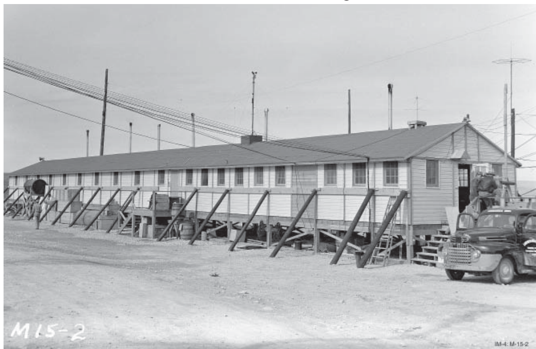
South side of the control point building. Entrance to the control room is at right. Men on porch are looking north toward ground zero. Note braces shoring up the building. Source: Los Alamos National Laboratory.
