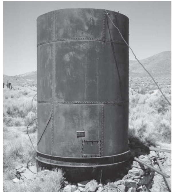
Tippihah Spring, top, with water storage tank made from a boiler. Source: DOE, Nevada Operations Office.
