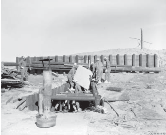
Workers repairing the blockhouse on January 31, 1951, following Baker. Note the protective masks and foot coverings. Source: Los Alamos National Laboratory.
