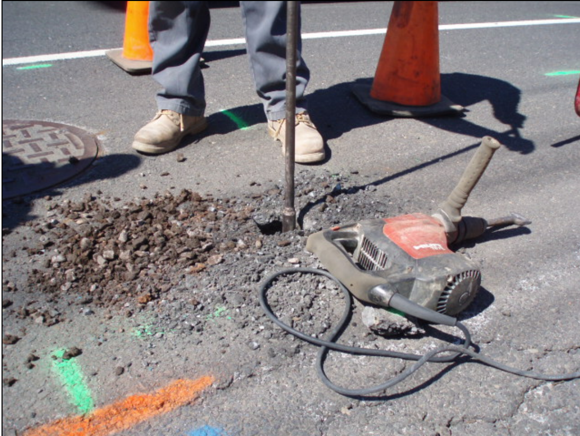
Fig. 2. Starting soil boring next to the manhole at the New Brunswick, NJ, Site.
