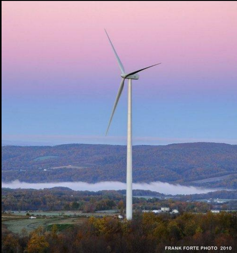
100 meter wind tower
