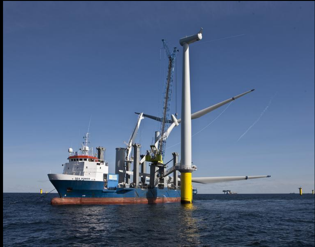
2.3 MW turbine: 93 meter diameter blades, 115 meters high.
