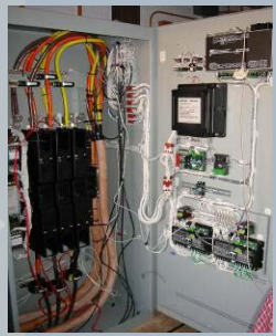
Switchgear, Relays, & Controls
