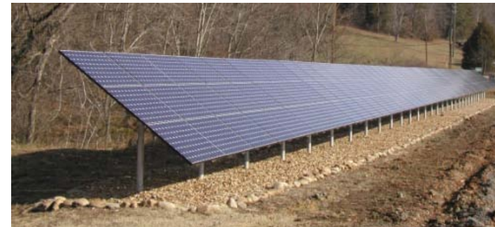
50kW PV Array is connected to the DECC Lab
