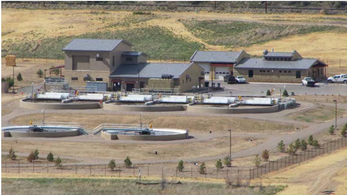
Figure 4. Photo of City of Rifle Wastewater Treatment Plant (taken May 3, 2010)
