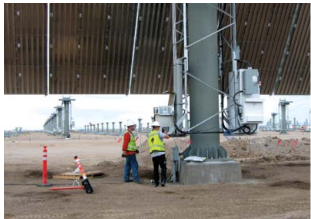
Workers testing the automatic stow-capability trackers for a concentrating solar photovoltaic module at the 30 MW Cogentrix solar power plant in Alamosa, Colorado.
