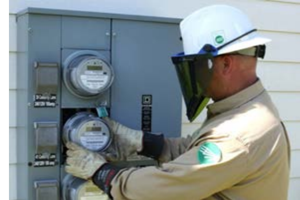
Technician changes out analog meter with a smart meter
