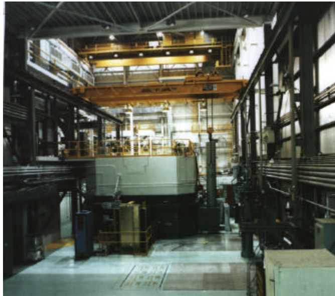
Figure 7. Transient Reactor Test Facility (TREAT) at Argonne National Laboratory (West)
