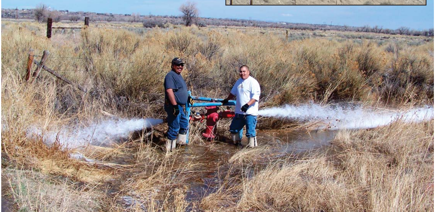
Hydrant flushing conducted by the Northern Arapaho Utility Organization.
