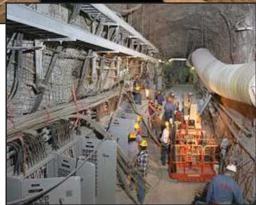
Scientific testing inside the tunnels of Yucca Mountain.
