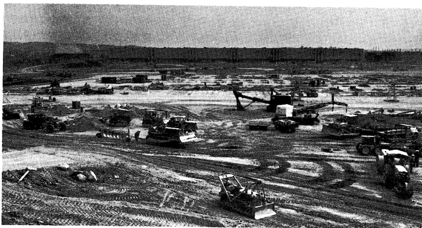
CONSTRUCTION AT OAK RIDGE, 1952 / Grading is in progress on the site of the new K-33 gaseous-diffusion plant as part of the Commission's expansion of production facilities. Other diffusion plants are in the background.
