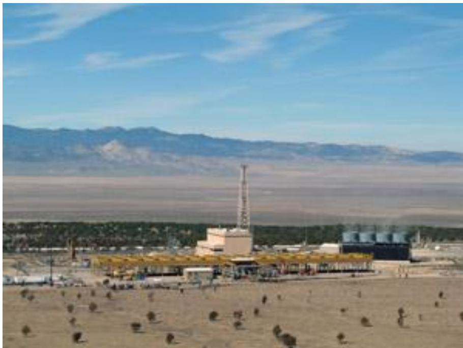
Blundell Power Plant Flash plant with binary bottom cycling unit
