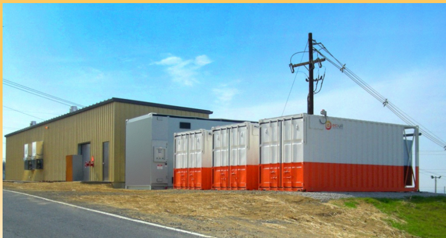
The PJM Interconnection regulation services project in Lyon Station, Pennsylvania.
