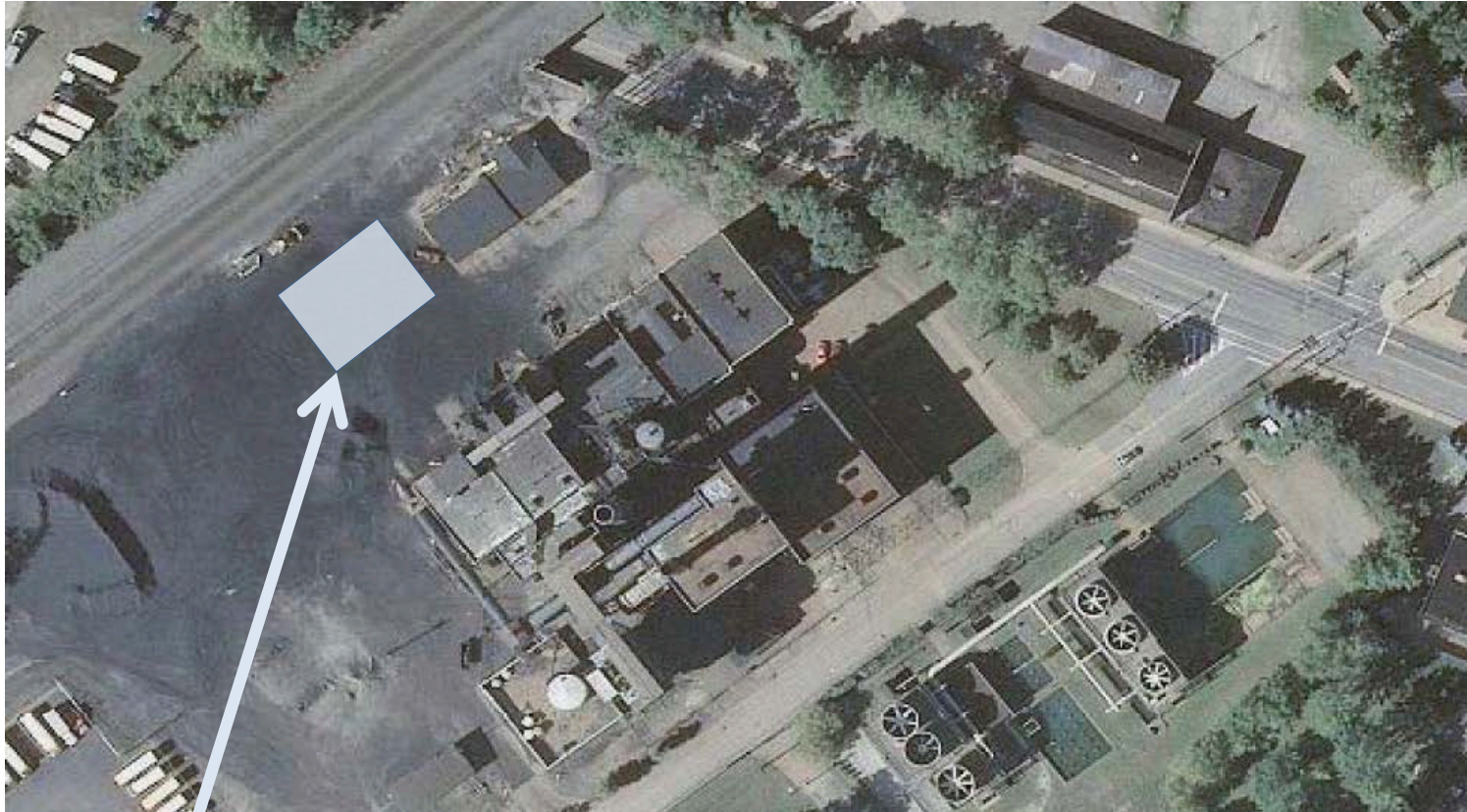
Battery Building Site
