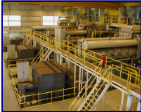
Port Allen Power Plant
