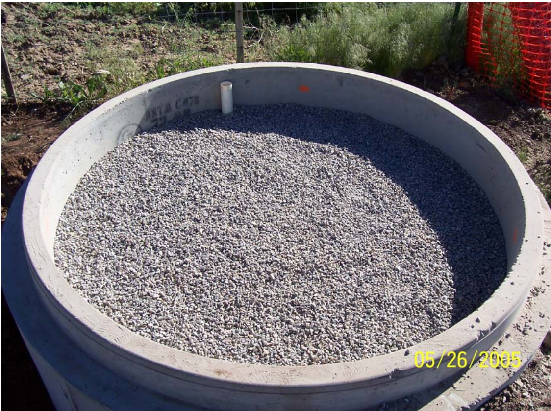
Figure 24. Top of Unit ; gravel covers the collection piping.
