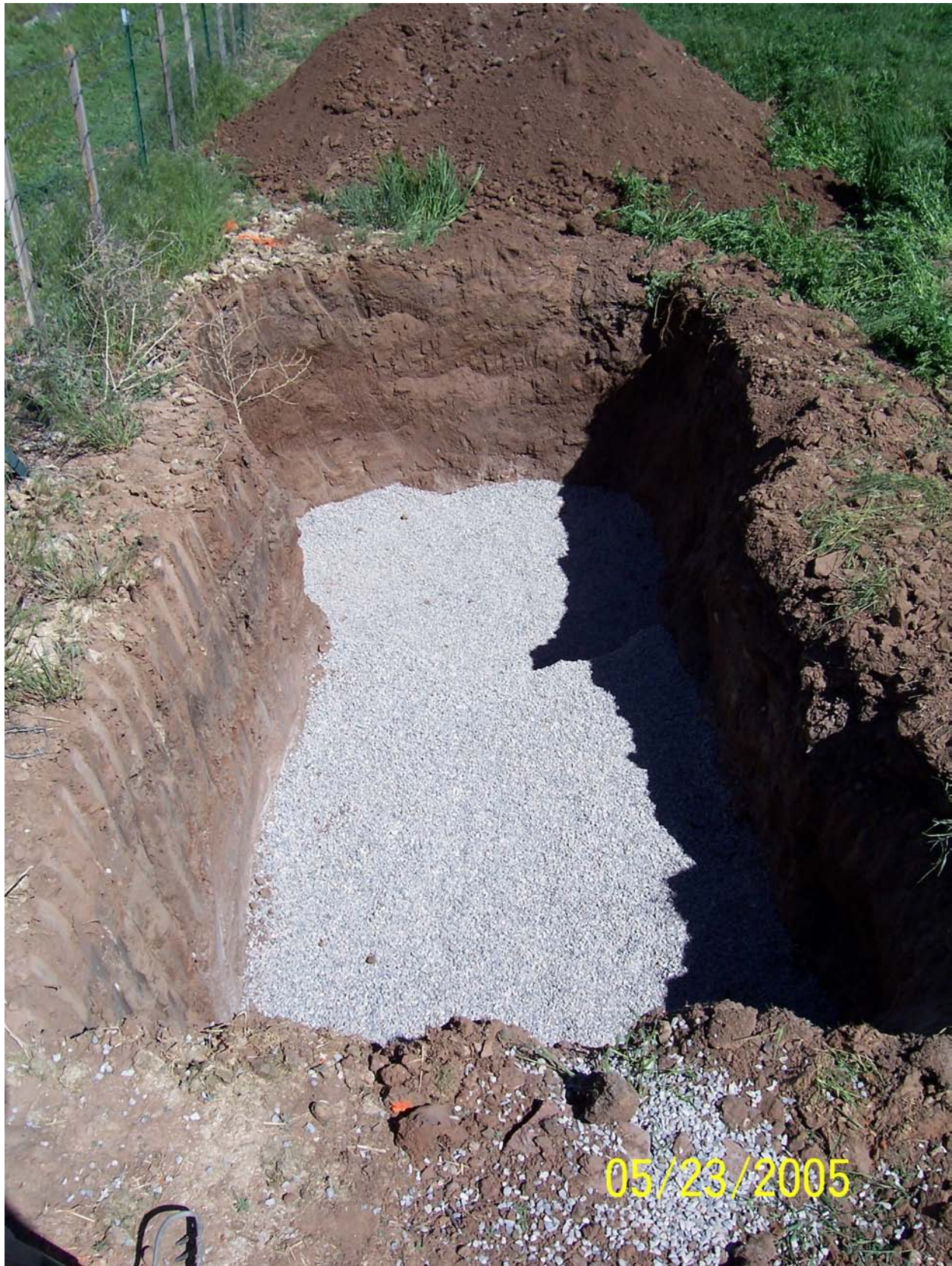
Figure 5. Excavation ready for treatment cell and valve box. Bed of pea gravel for leveling.
