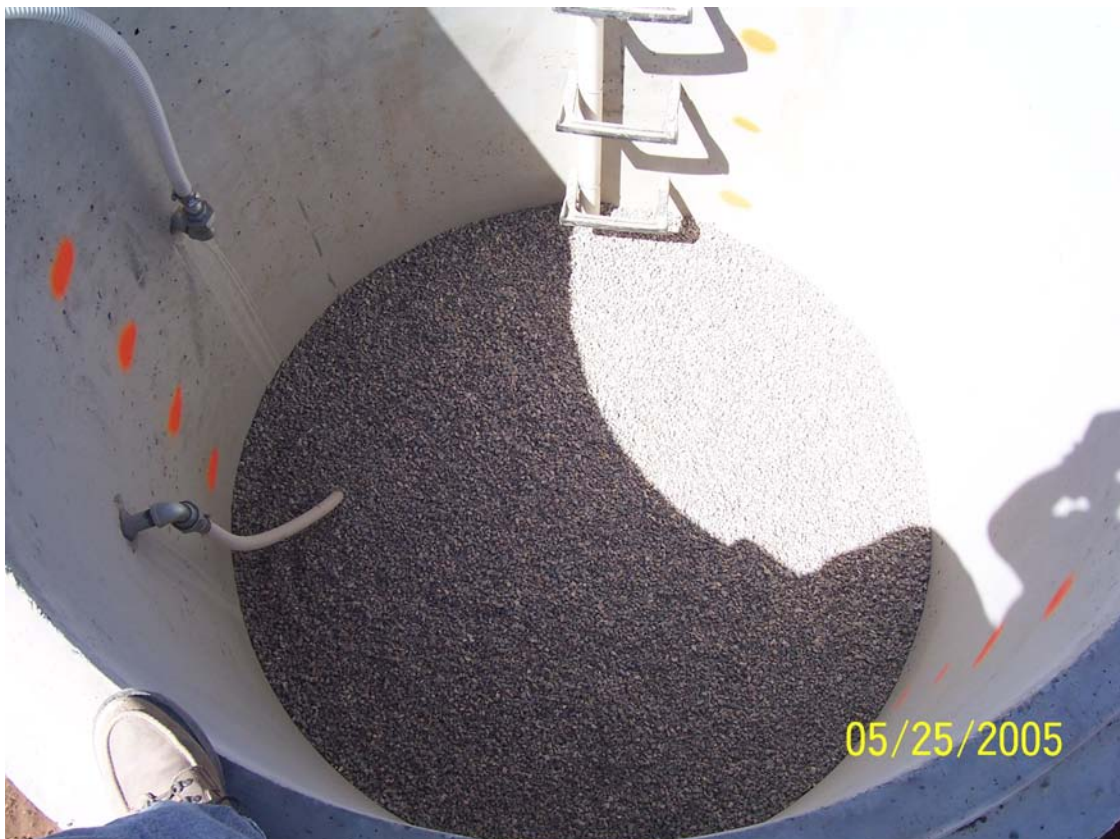
Figure 17. Treatment cell after installing Unit 1 (pea gravel and distribution piping).
