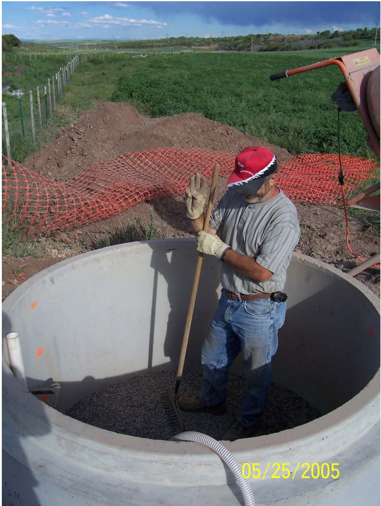
Figure 20. Top of Unit 3 after raking to homogenize.
