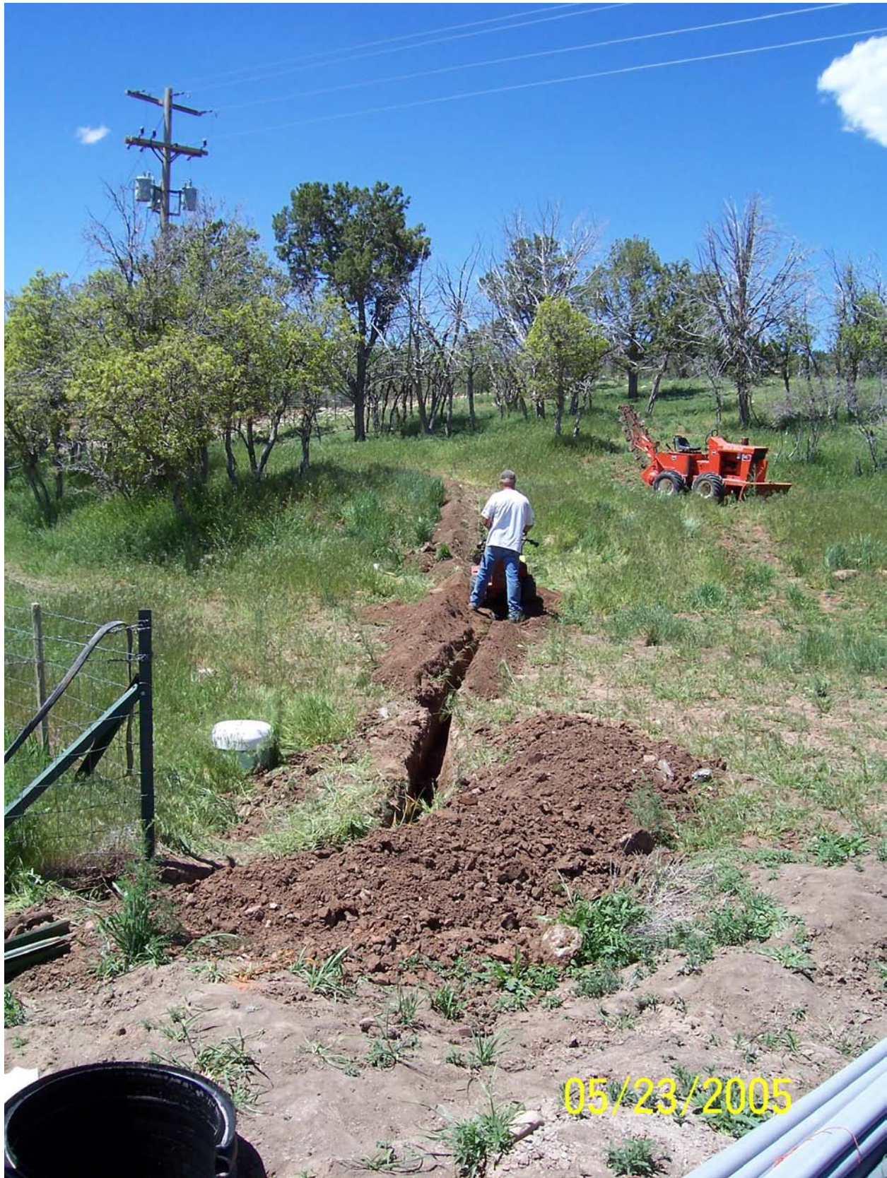
Figure 34. Trenching for electrical line to landowner's pump house. Electrical supply pole in background.
