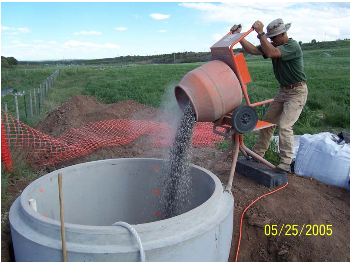
Figure 19. Gravel/ZVI mixtures were poured directly into the treatment cell, then raked to homogenize.
