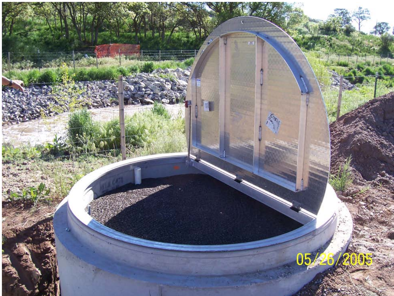
Figure 26. Treatment cell filled with reactive material with aluminum lid in place. Note bar that keeps door in upright position and top of well.
