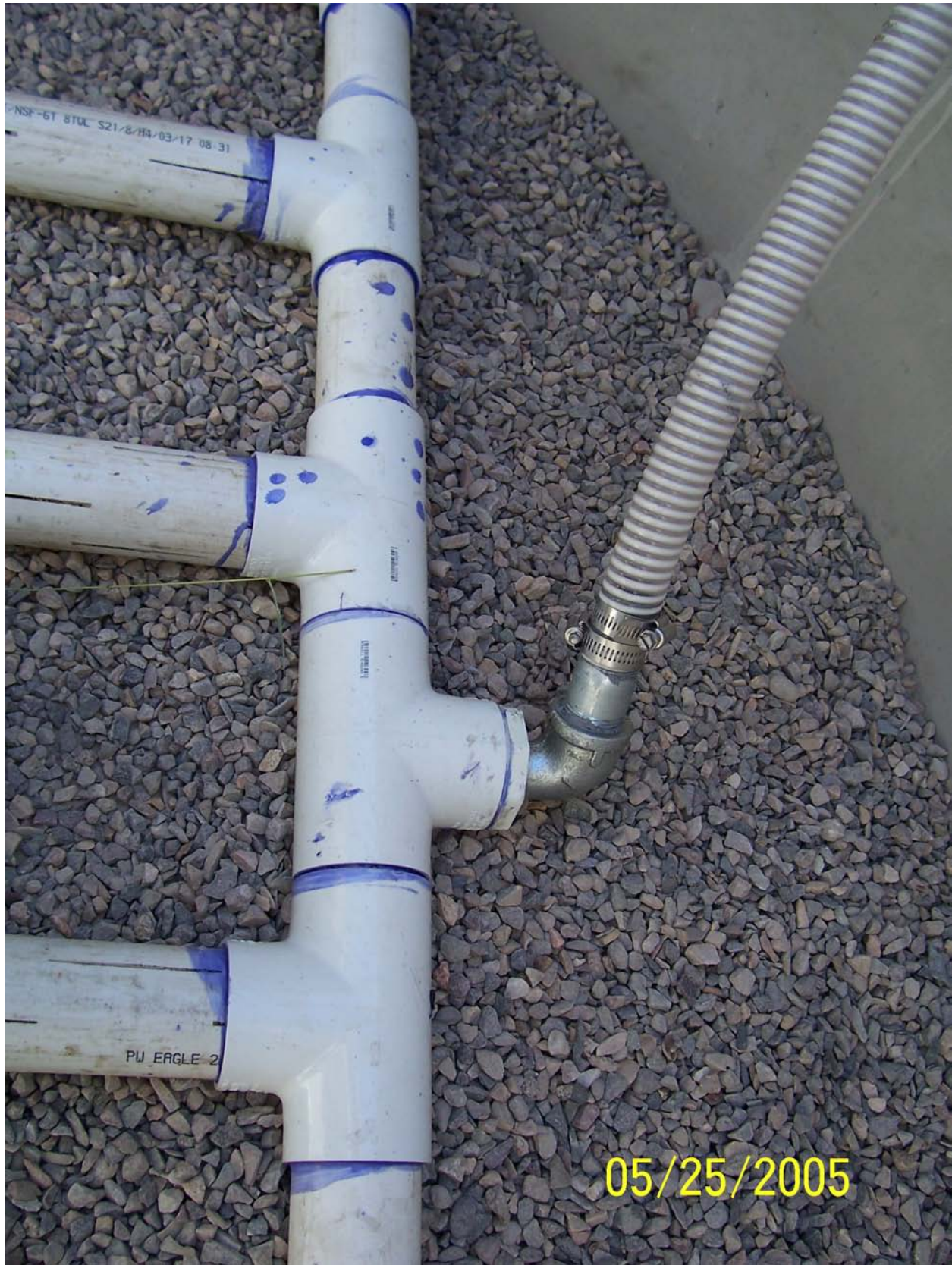
Figure 12. Galvanized connection from distribution piping to reinforced 1-inch flex hose.
