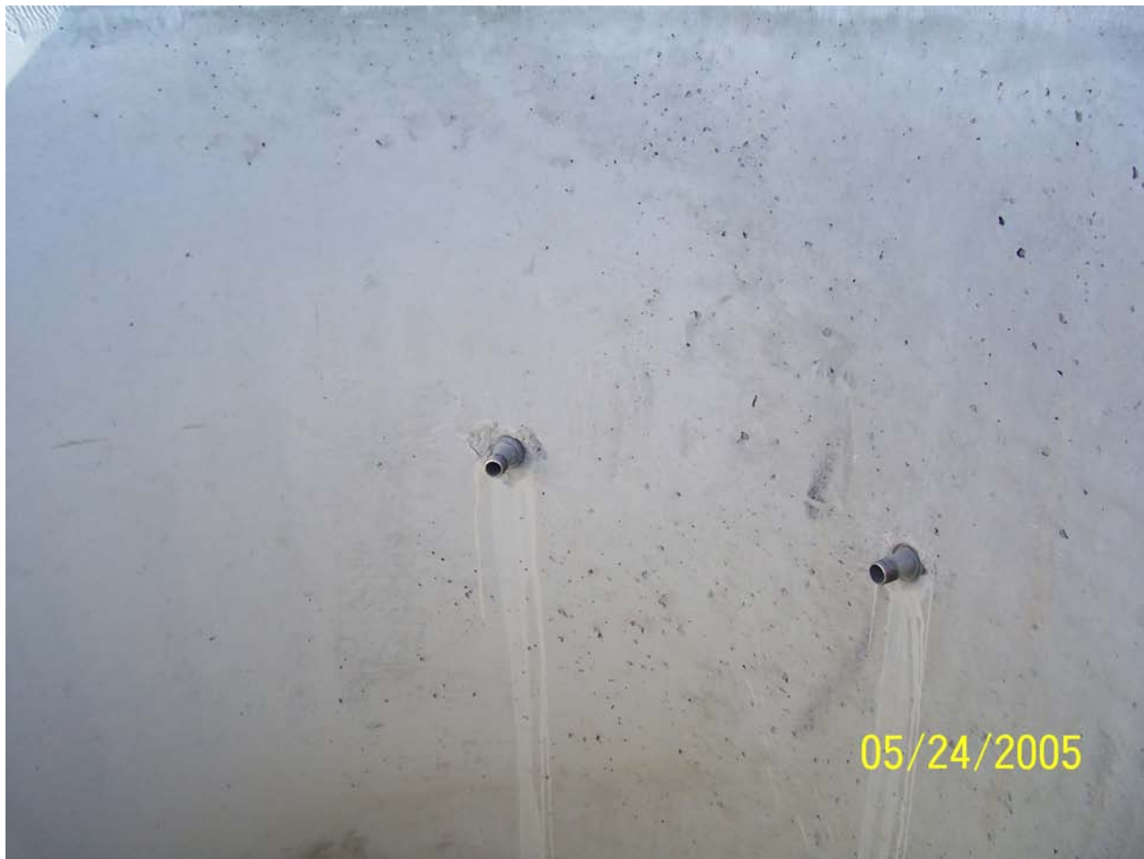
Figure 8. Galvanized nipples (1 inch) for connection to valve box from inside treatment cell.
