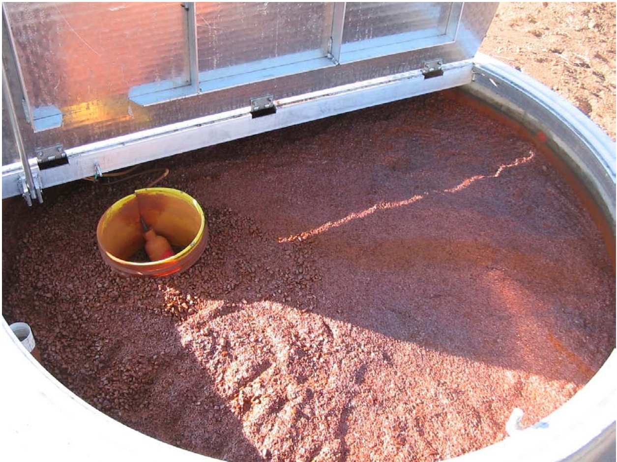
Figure 27. Float switch temporarily positioned in plastic bucket. The switch was later mounted permanently to the ribbing on the aluminum lid. Note the red rust color of the ZVI layer, this photo was taken about 2 weeks after startup.
