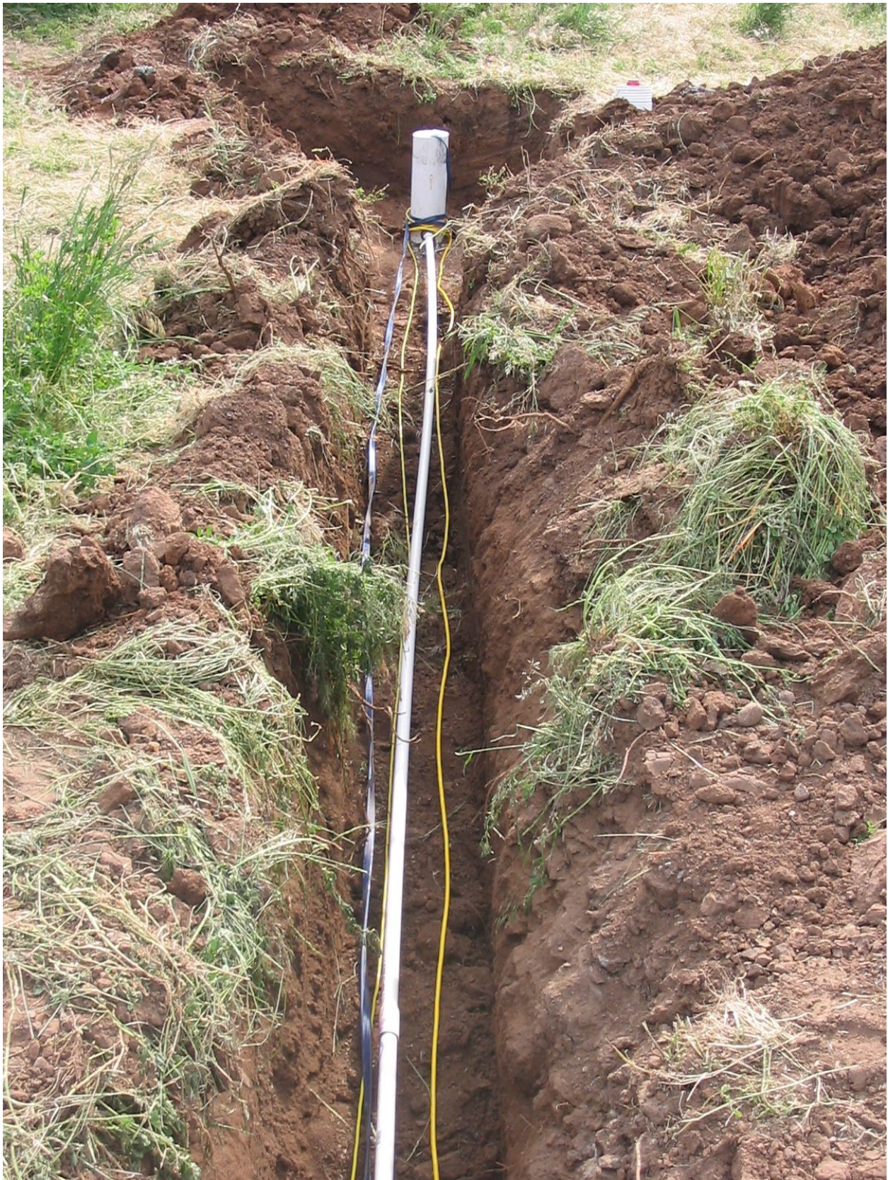
Figure 35. Piping (1-in schedule 40 PVC) and cables going to extraction well EW-1 prior to burial. Blue cable is 220 volt power for pump. Yellow cables are connections for level sensors and transducer signal.
