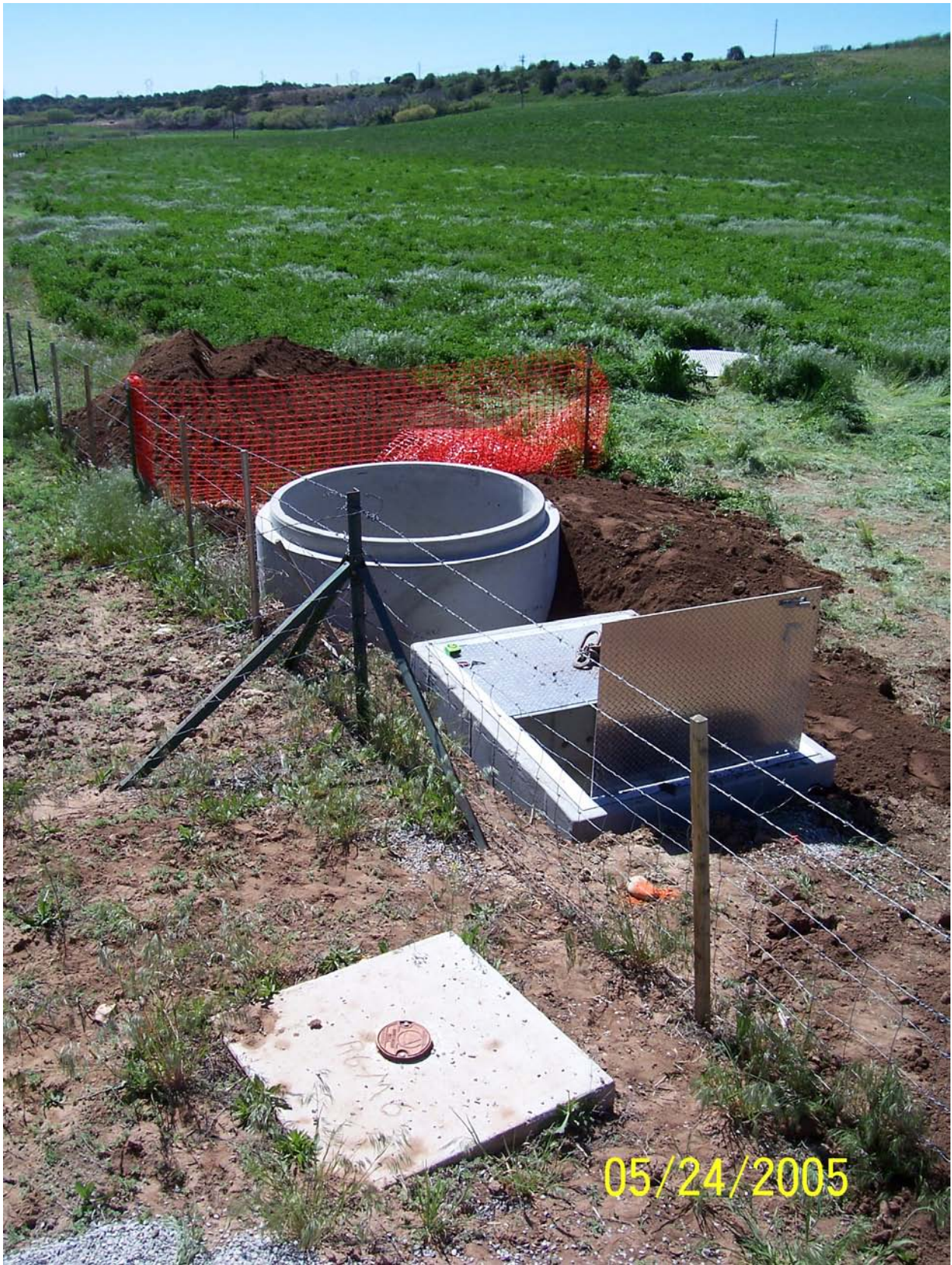
Figure 3. Placement of valve box and treatment cell
