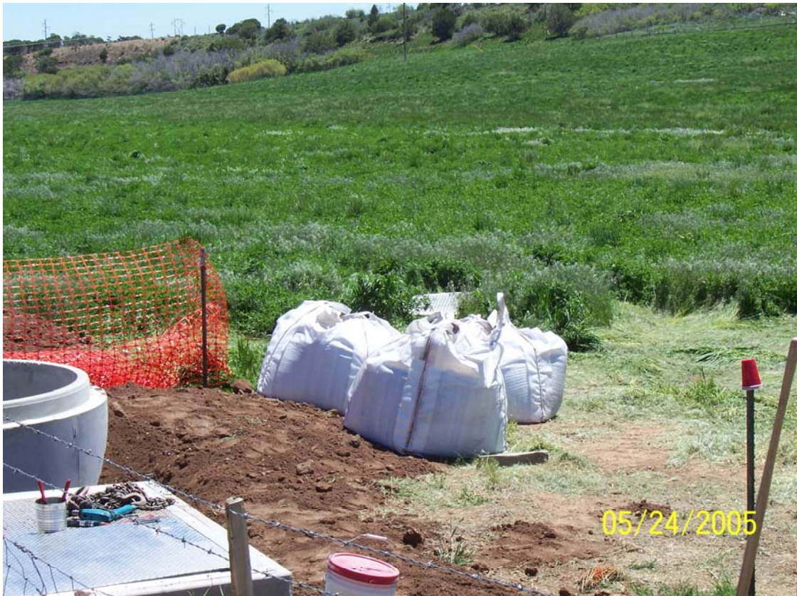
Figure 16. Zero-valent iron in super sacks. Each sack contains 1 ton of -4 +10 mesh ZVI. Two tons were used in treatment cell (one additional bag of ZVI was ordered and delivered but not used).
