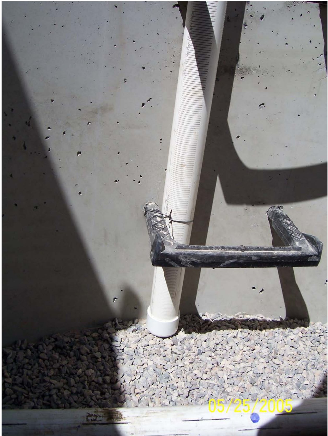
Figure 10. Bottom of well in treatment cell resting on 2-inches of pea gravel. Distribution pipe in foreground.
