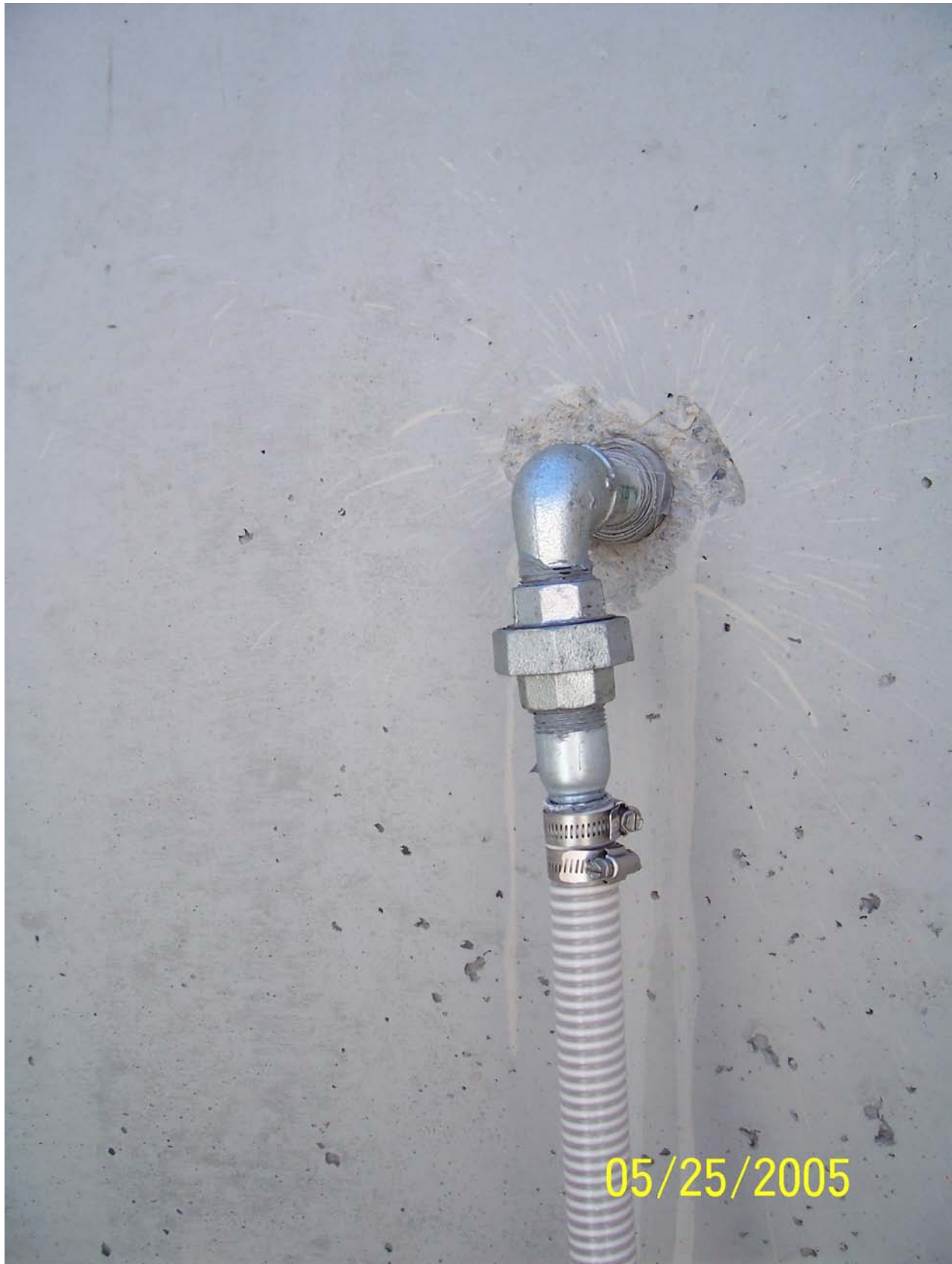
Figure 11. Galvanized connection with union from reinforced flexible hose coming from distribution piping to 1-inch-threaded galvanized nipple coming from valve box.
