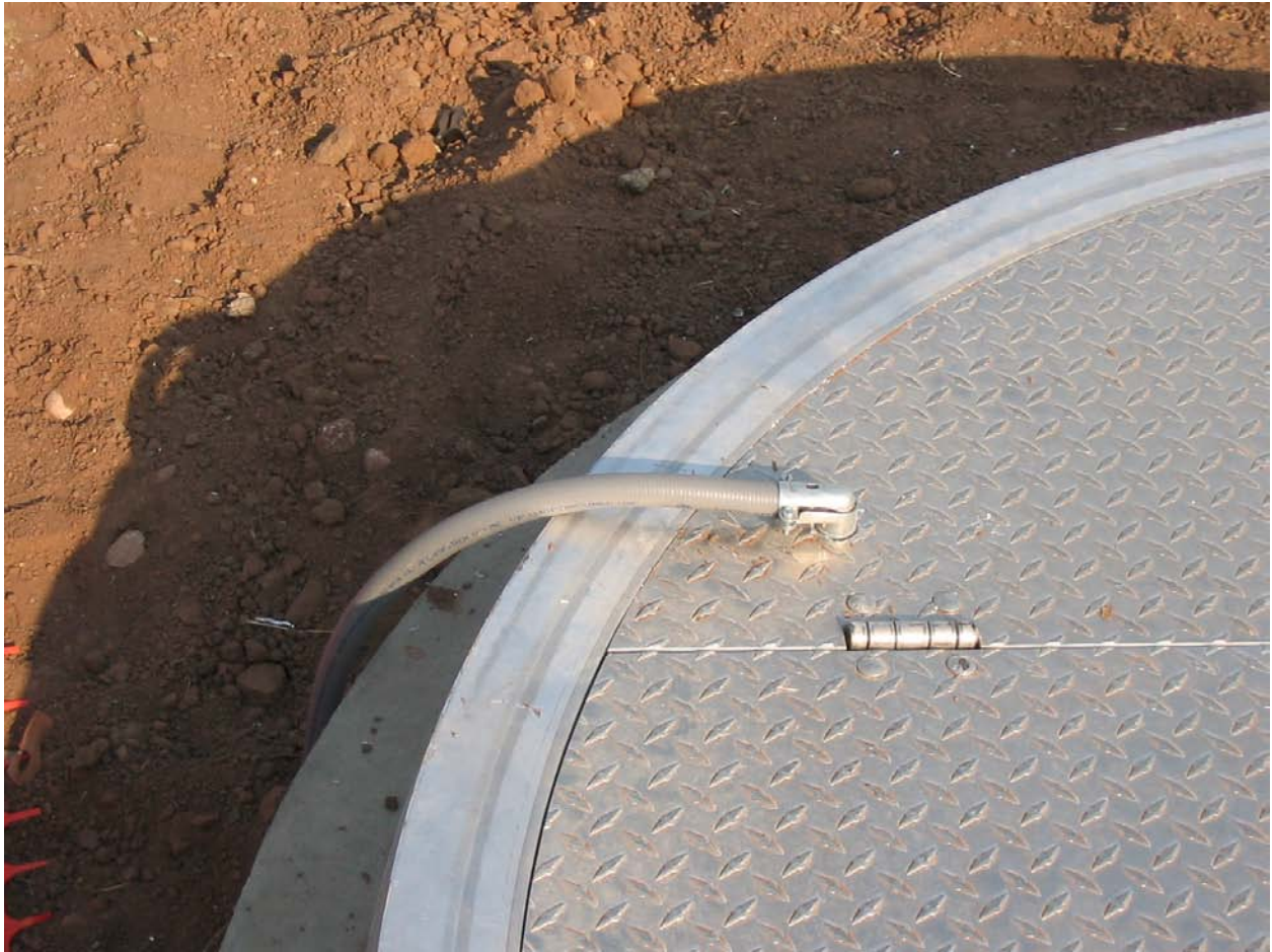
Figure 28. Electrical connection for float switch on top of treatment cell lid.
