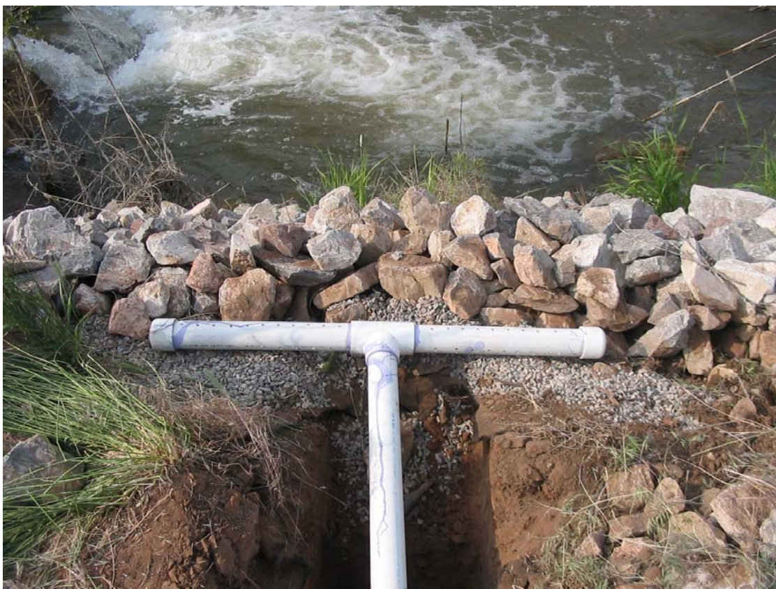
Figure 39. Infiltration gallery before burial.
