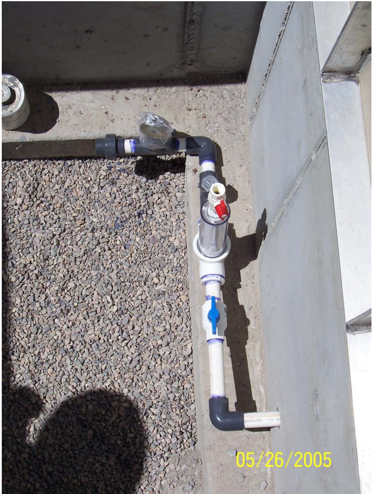
Figure 29. 1-inch PVC pipe outflow line passing through hole cut in east end of valve box.
