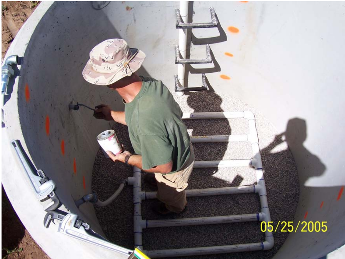
Figure 13. Distribution piping in place on 2-inch bed of pea gravel. Orange paint marks at 1-ft intervals from base of concrete treatment cell.
