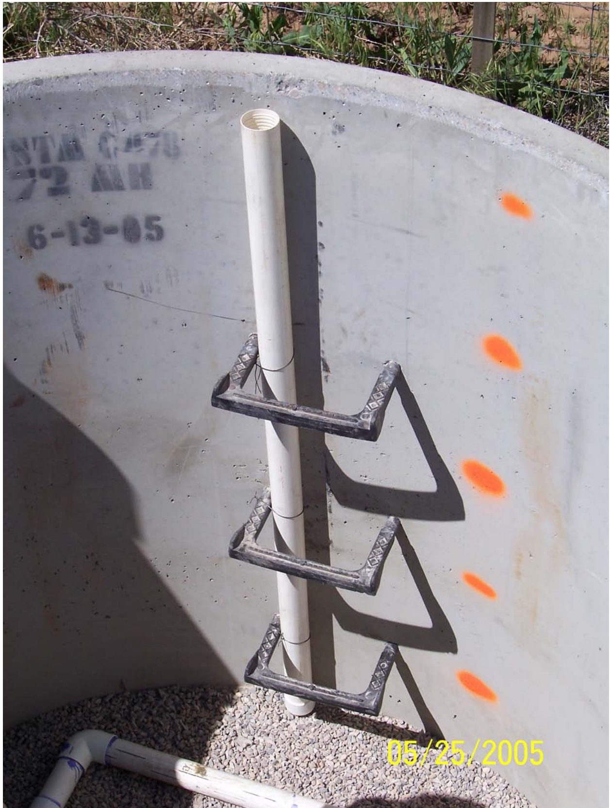
Figure 9. Well in treatment cell. Two-inch-schedule 40 PVC pipe with slotted well screen and end cap. Orange paint marks are at each foot from base of treatment cell.
