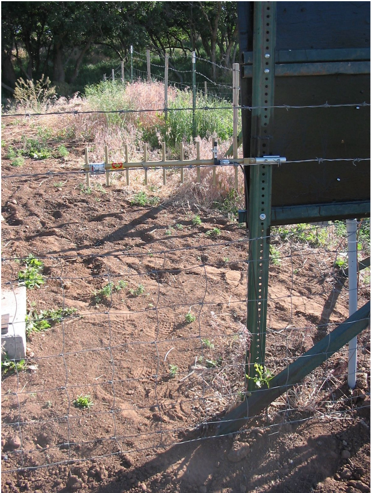
Figure 32. Antenna for data transmission. Attached to electrical panel.
