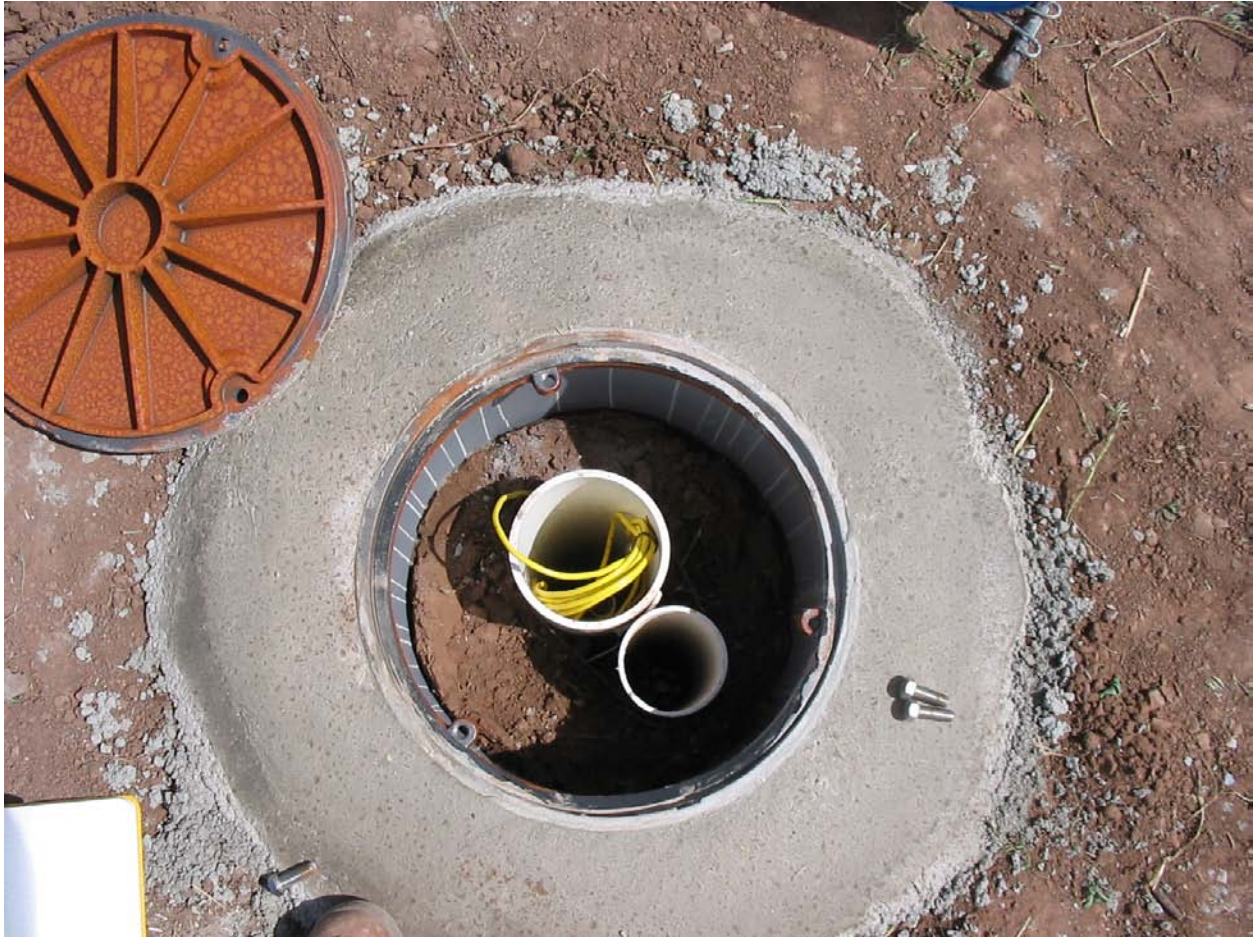
Figure 43. Completed well IW-1. Small PVC pipe is valve riser. Yellow cable is for transducer.
