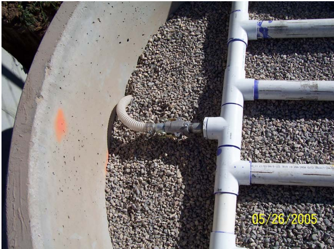
Figure 22. Camlock connection of collection piping to flexible hose.
