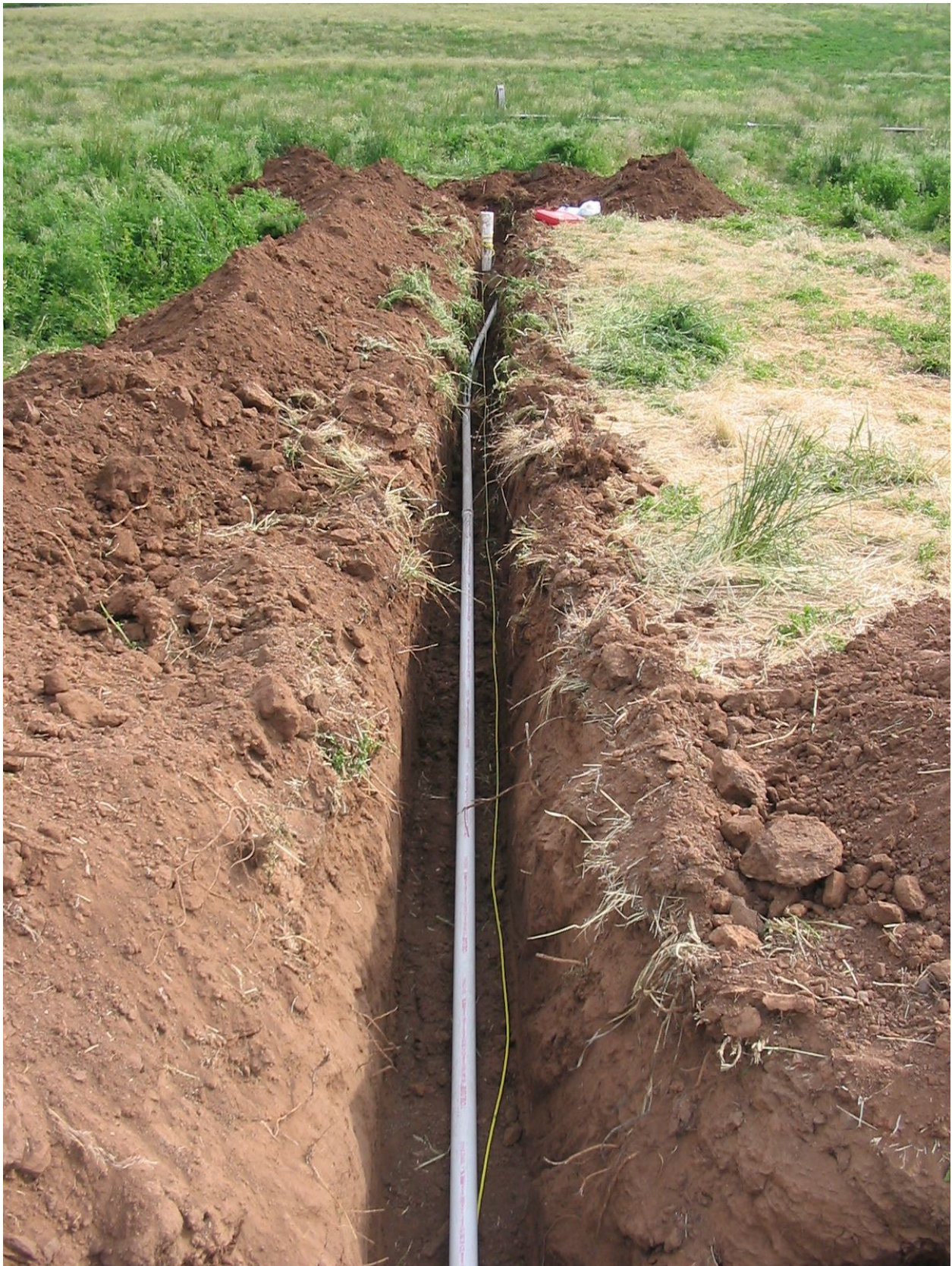
Figure 37. Piping (2-inch schedule 40 PVC) and yellow transducer cable going to well IW-1 prior to burial.
