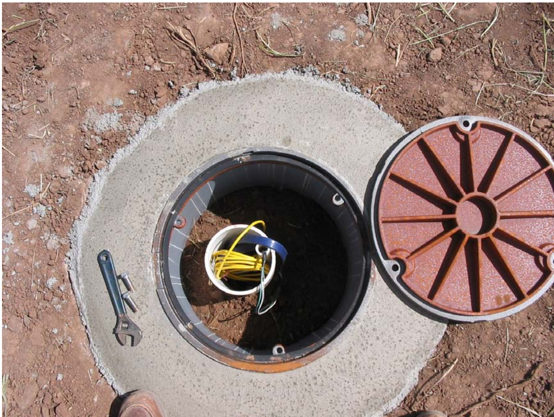
Figure 42. Completed well EW-1. Small (0.5-inch) internal PVC pipe houses the water level control sensors. Yellow cable is for transducer. Blue cable is 220-volt power supply for pump.
