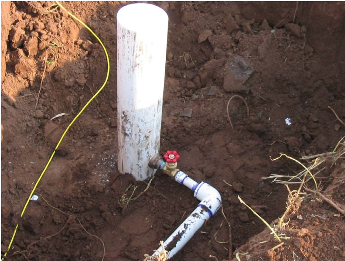
Figure 38. Connection to IW-1 showing pitless adapter and gate valve.
