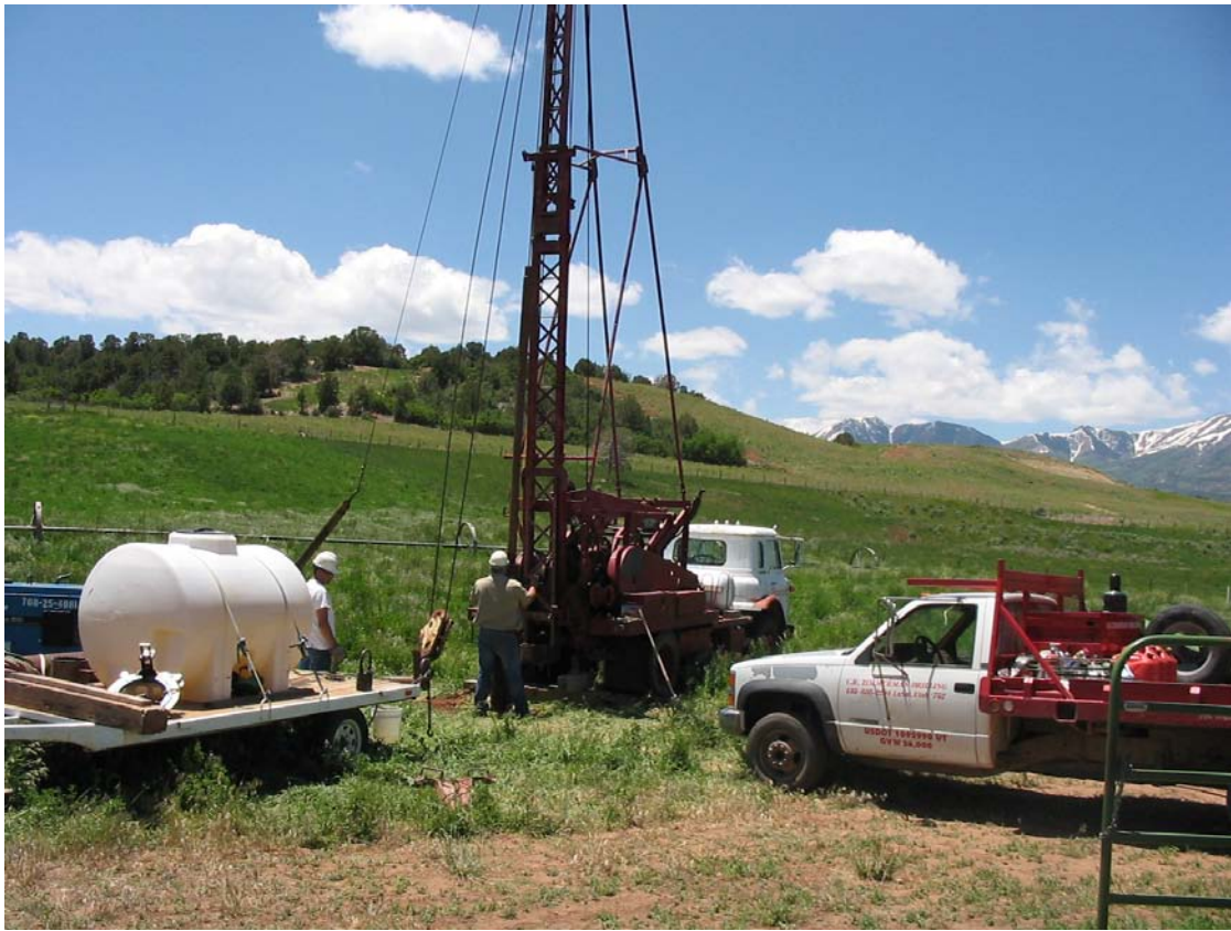
Figure 41. Cable tool drilling rig set up on well EW-1.
