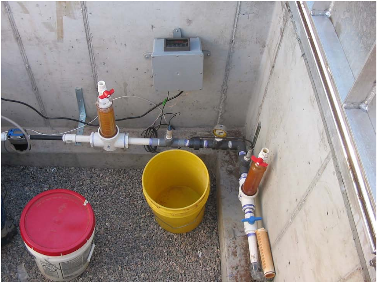
Figure 30. Portion of outflow line showing valve, filters, pressure transducer, pressure gauge, pH probe, and flow meter.
