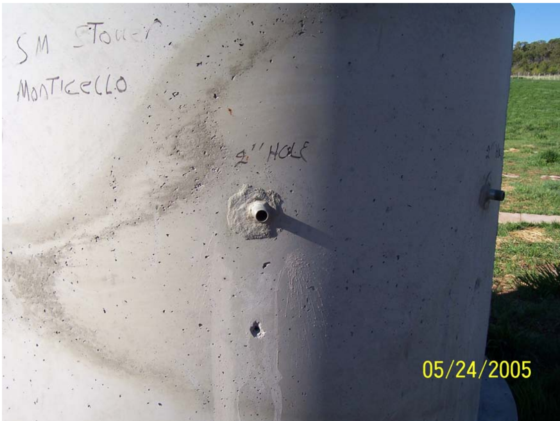
Figure 7. Galvanized pipe (1 inch) grouted in treatment cell for connection to valve box.
