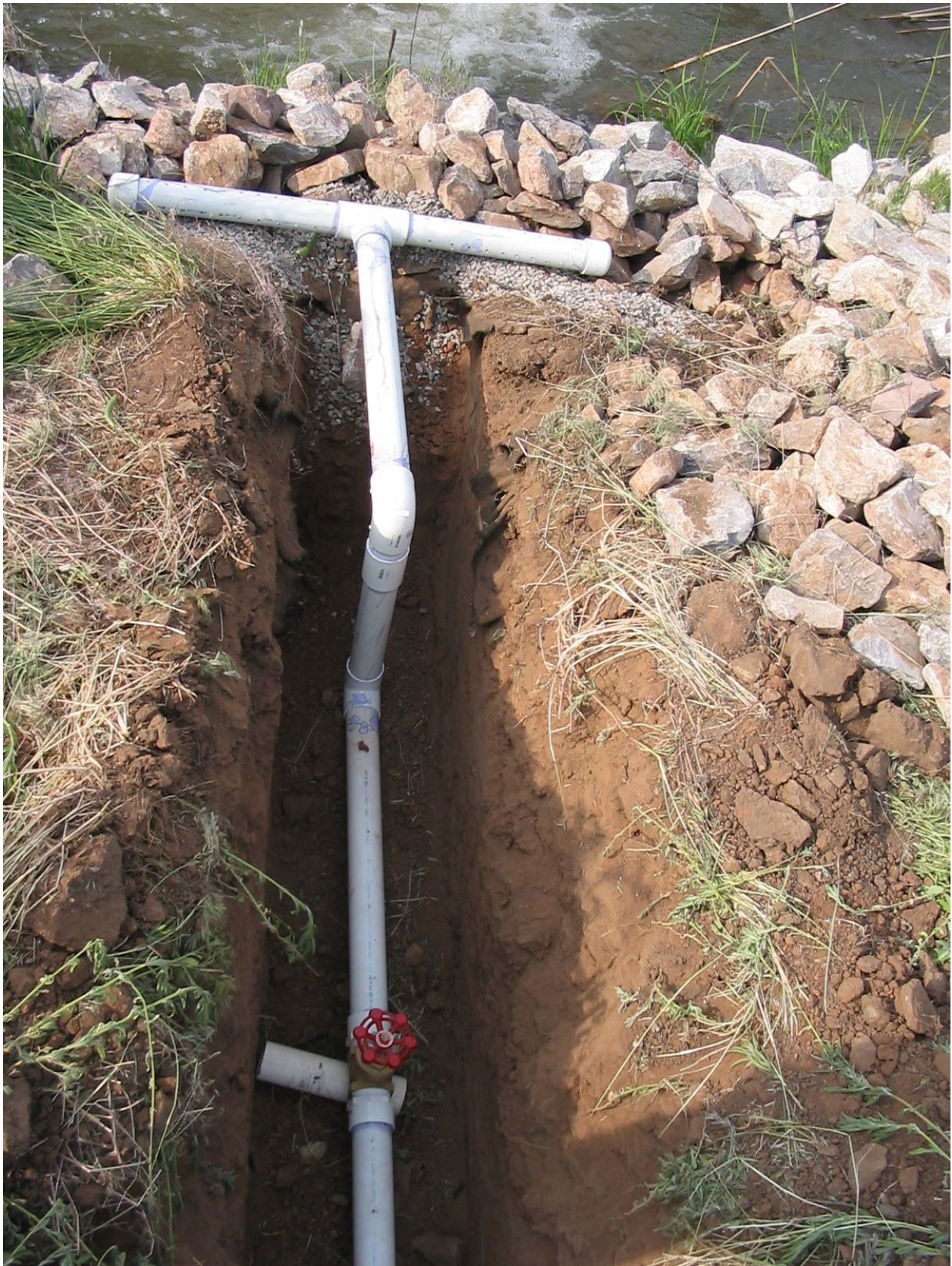
Figure 40. Gate valve and riser to infiltration gallery.
