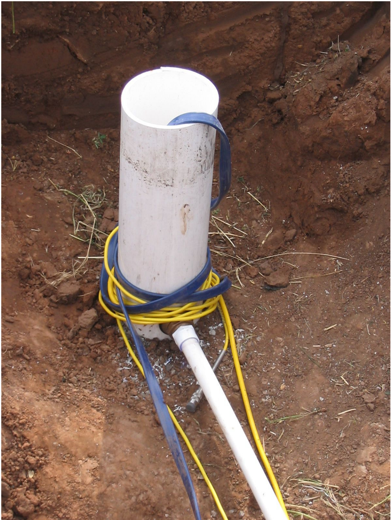
Figure 36. Closeup of pipe and cables at well EW-1 showing pitless adapter.
