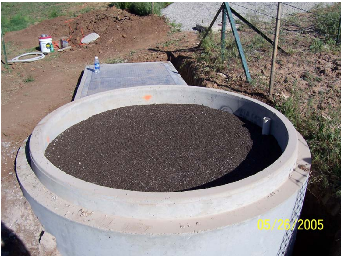
Figure 25. Top of Unit 6 (ZVI). Filling of the treatment cell is complete. Orange paint mark is 5 ft from base of the concrete floor.
