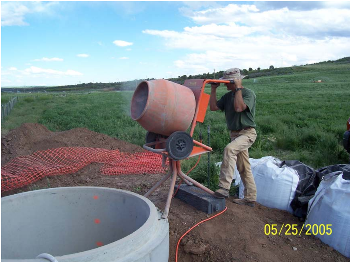
Figure 18. Mixing pea gravel and ZVI in a concrete mixer.
