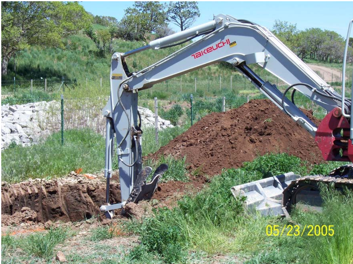
Figure 4. Excavation for treatment cell and valve box.
