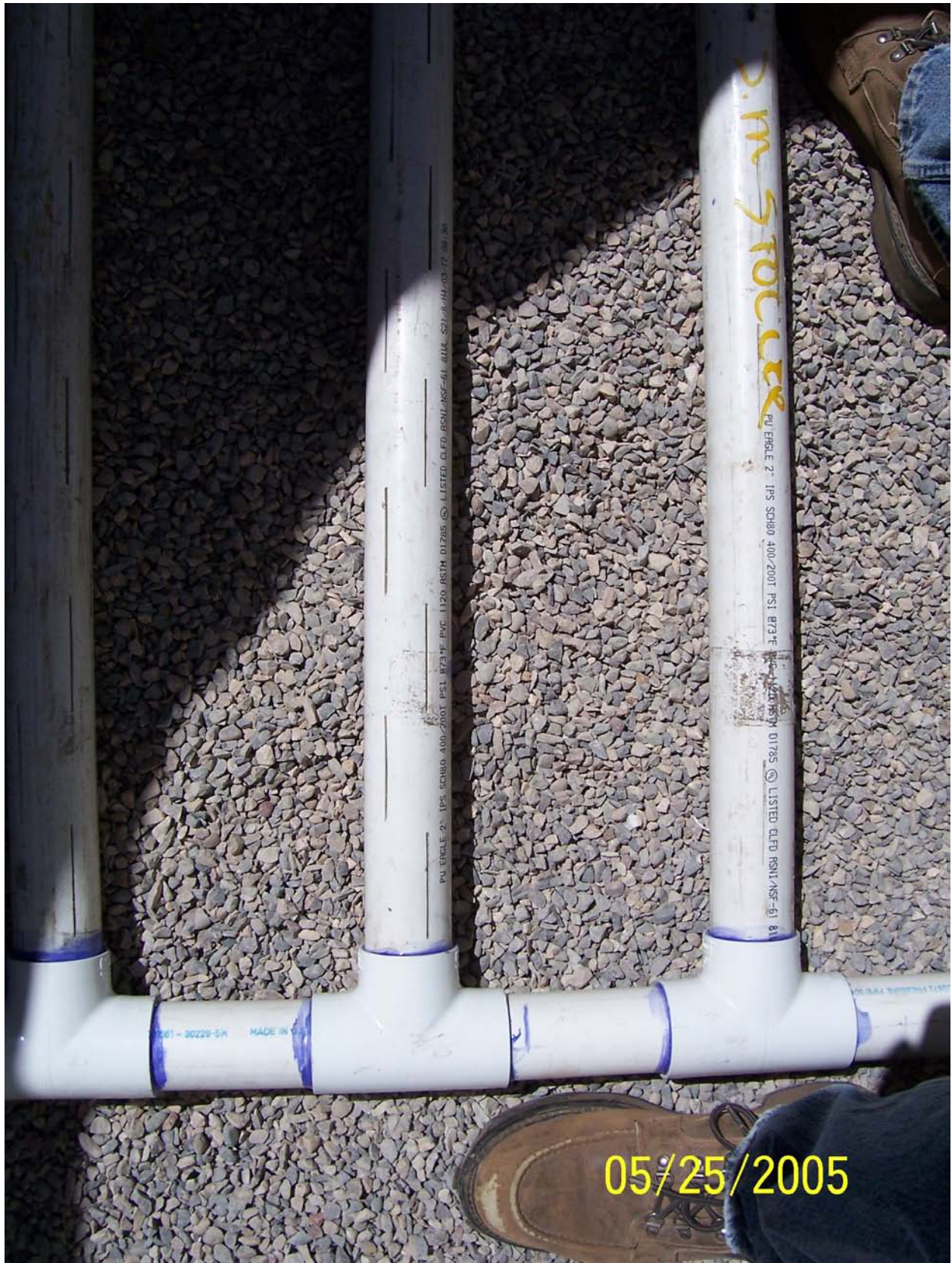
Figure 15. Close up of PVC connections in distribution system.
