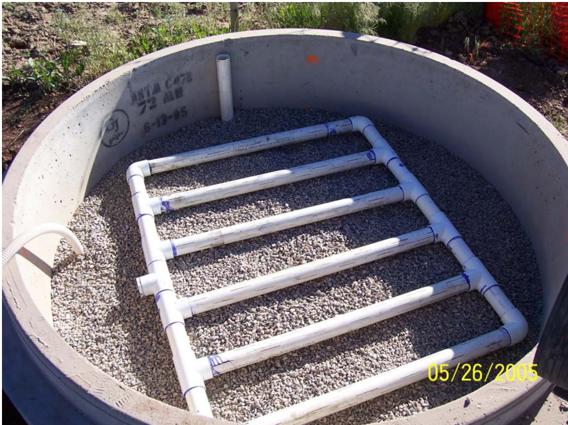
Figure 21. Collection piping system (Unit 5) resting on about 2-inch thickness of pea gravel.
