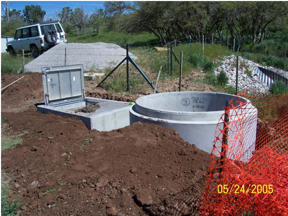
Figure 6. Treatment cell and valve box in position. Pea gravel pile in background.
