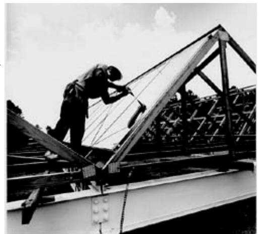
Dedication of the nation's largest solar heating and cooling system, currently in operation, took place November 26, 1975, at the George A. Towns Elementary School in Atlanta, Georgia. Solar collector panels mounted on the roof are pictured during construction.
