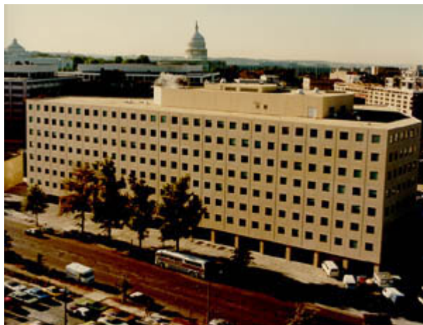
ERDA Headquarters, 20 Massachusetts Avenue, NW, Washington, DC, Summer 1975.
