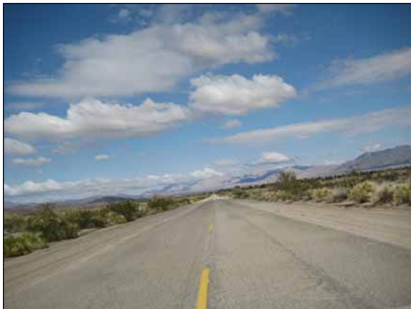
Figure 3.15-6 Photograph of Kaiser Road One Mile North of SR 177 Looking North
