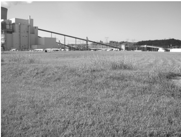
Figure 3.8-2. Proposed CO 2 Capture Facility Site
