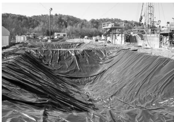
Figure 2-18. Lined Mud Pit
