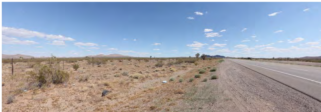
12 Figure 3.9-4. KOP 2 – View from US-95 Looking Southwest
