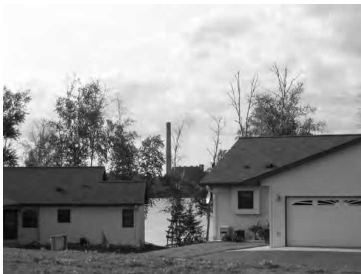
Figure 4.11-1. View of Syl Laskin Plant from Residences on Colby Lake
