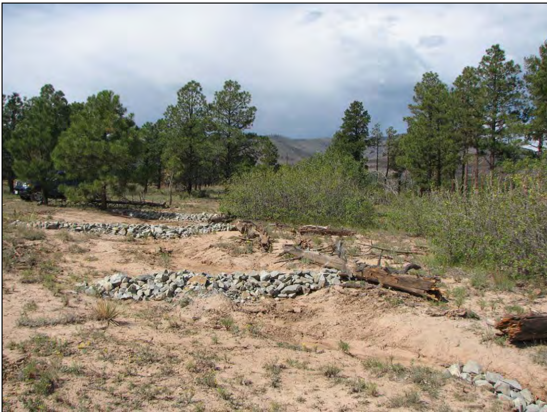
Figure 12. New rock erosion-control measures, LA 21334 (2011).
