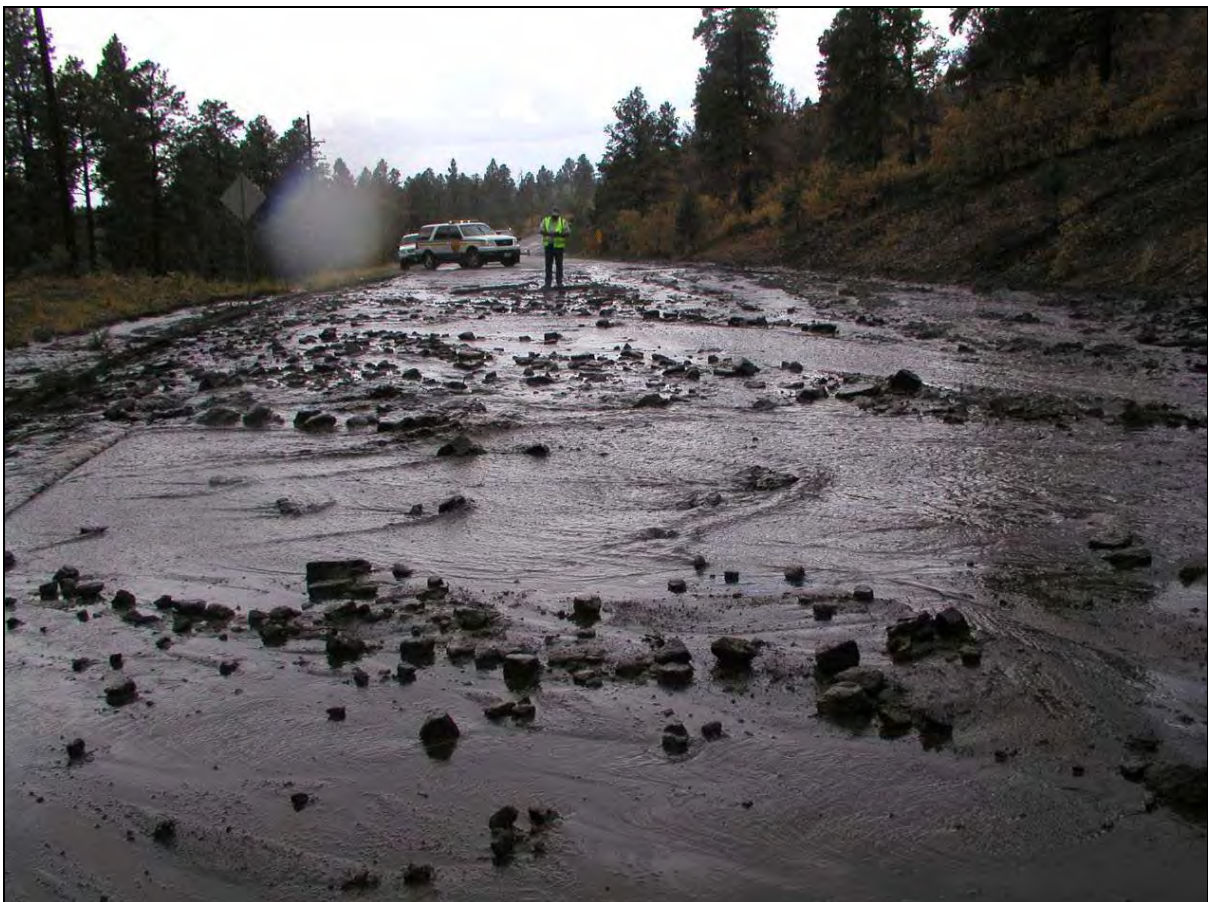
Photograph 36. Post-fire flooding effects on NM 501.
