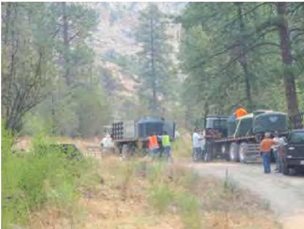
Photograph 10. Crews remove sediments and waste from canyon.
