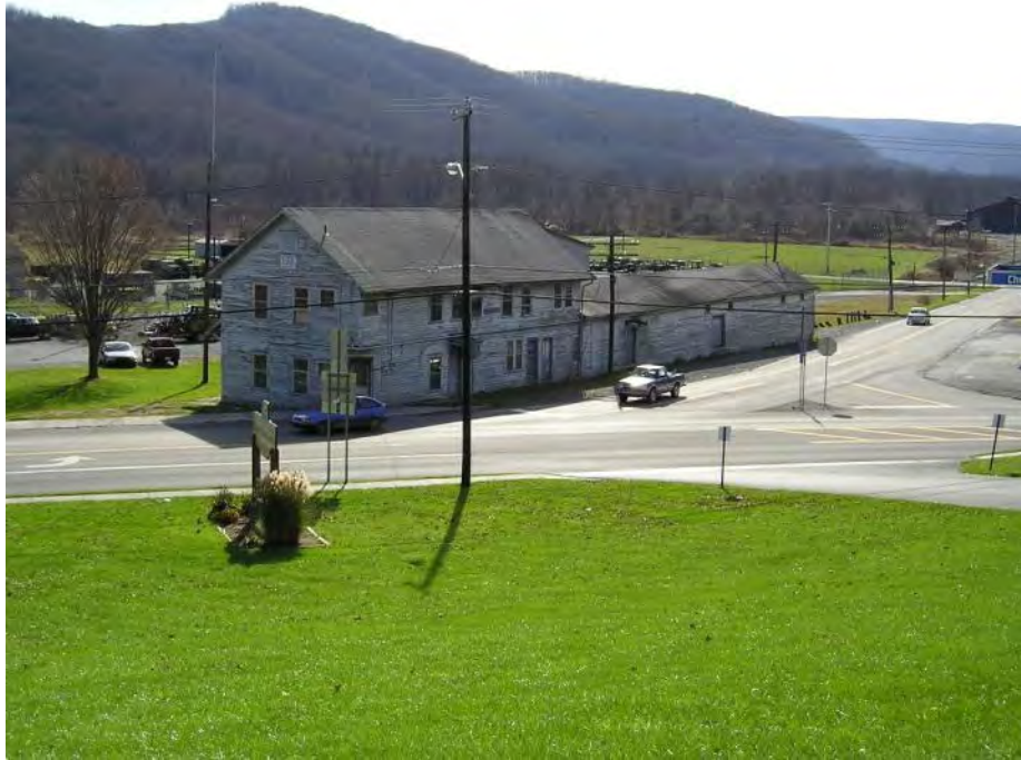
Figure 3.2-4. View toward Project Site at Intersection of US 60 and WV 20, Facing South
