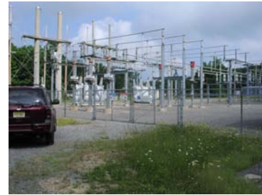
Grassy Falls Substation
