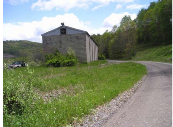
Figure 2.2-12. View of DN1
