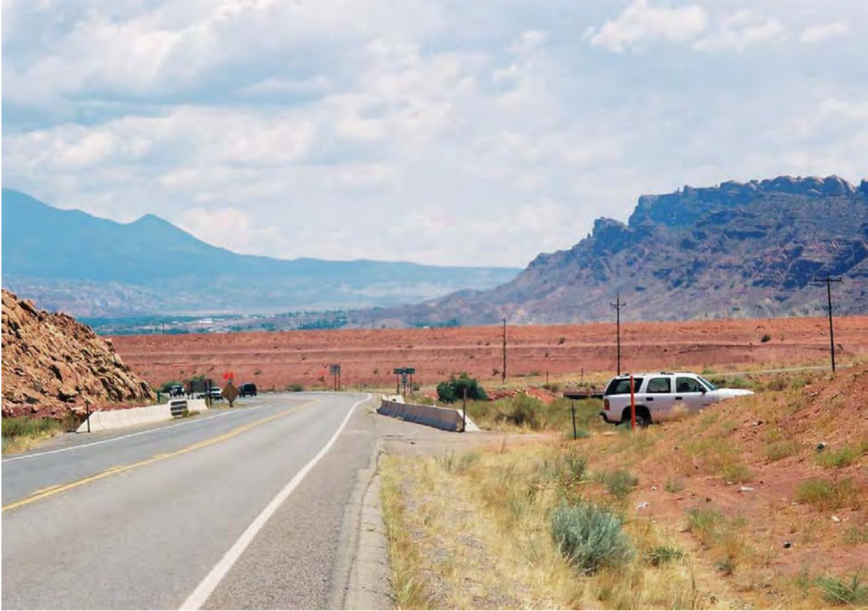
Figure 3–20. View of the Moab Site Tailings Pile from Southbound US-191 [Before UDOT widened US-191]
