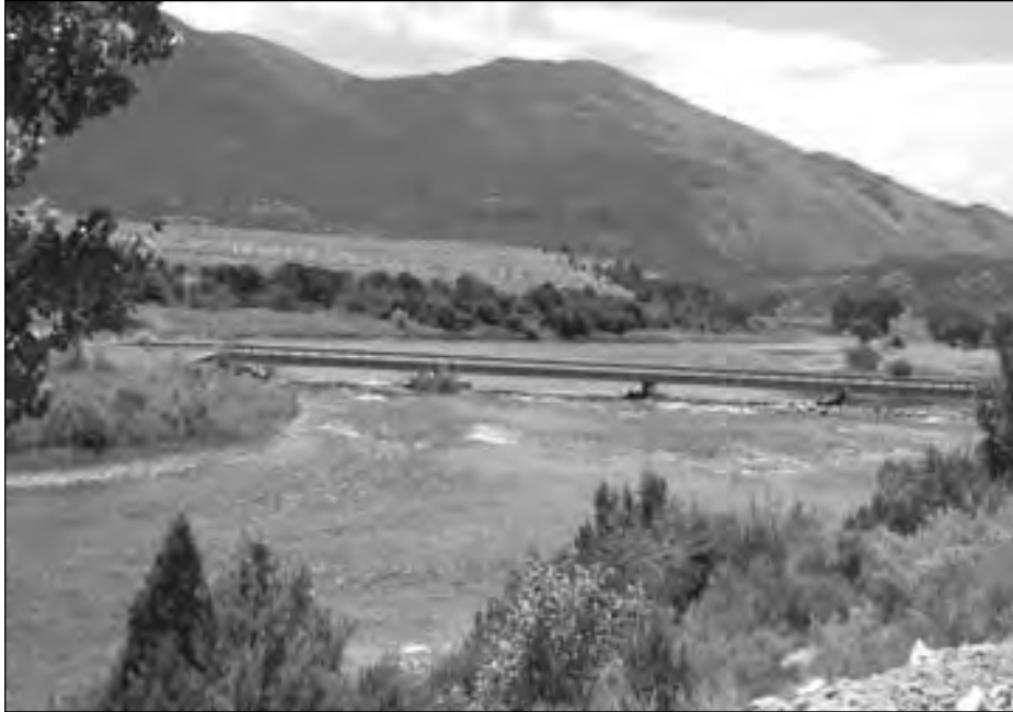
Looking North at Brown's Park Bridge.
