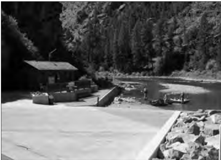
View of Green River from Dam Spillway Launch Ramp.
