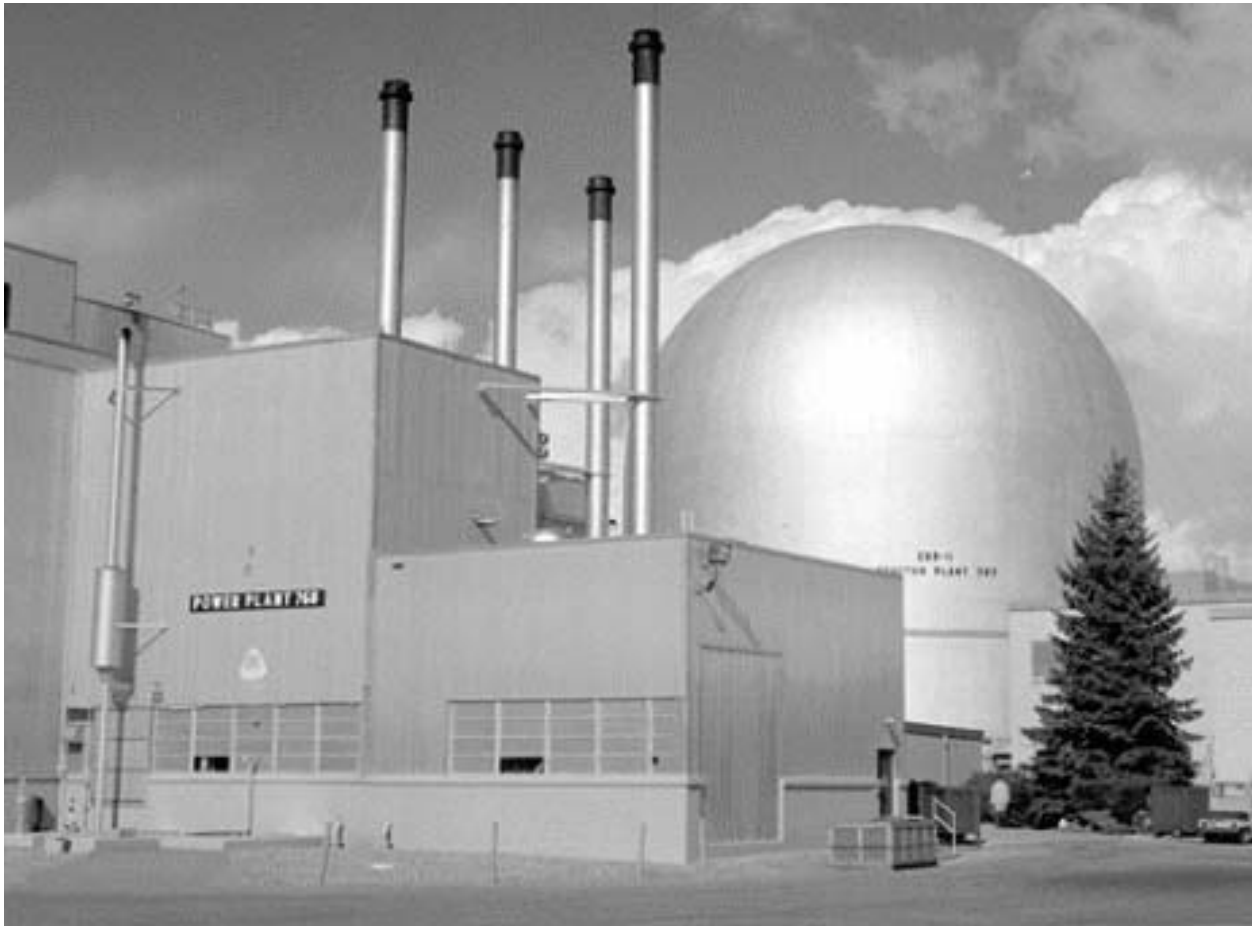
Figure S-16 EBR-II Facility
