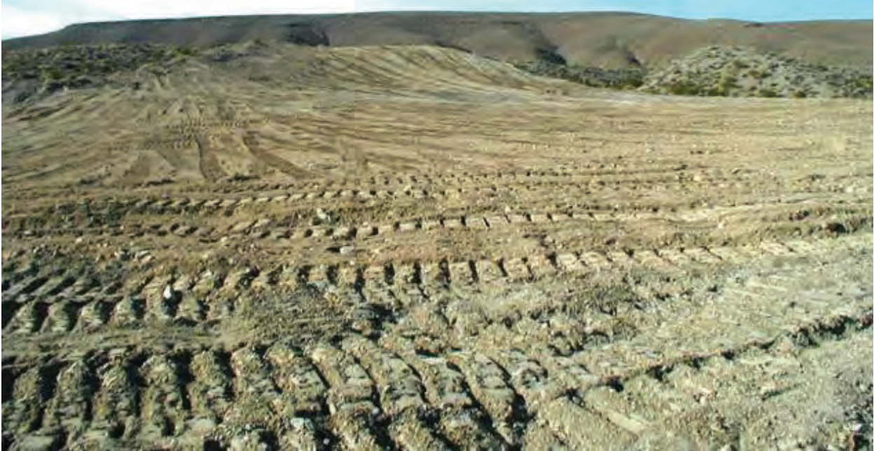
Figure 4-3. Decommissioned borrow area that has been recontoured prior to seeding and mulching.
