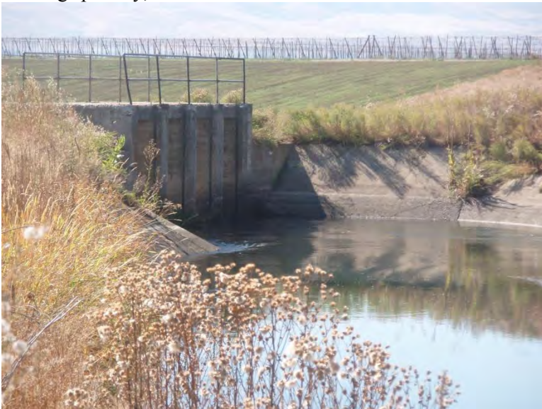
Upper portion of existing spillway view to southwest.
