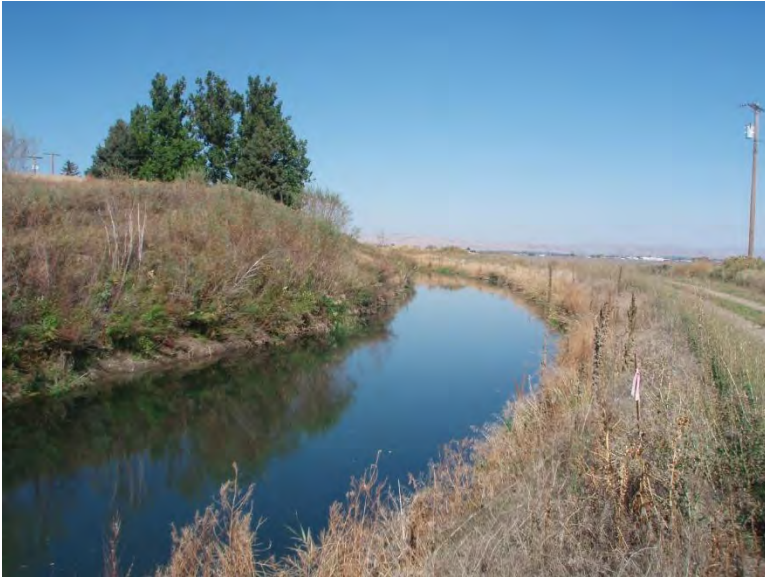
Main Canal above spill gate view to north.
