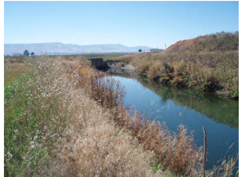
Main Canal view to southwest of spillway.
