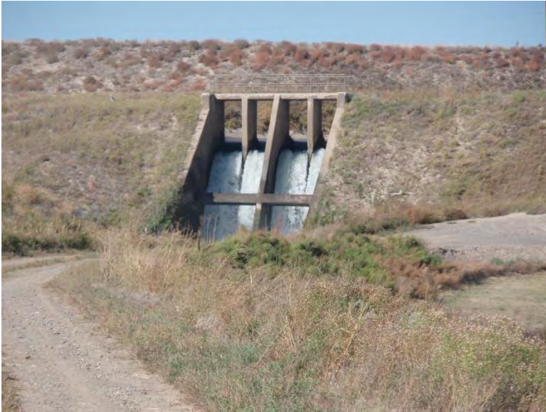
Existing spillway, view from southeast to northwest.
