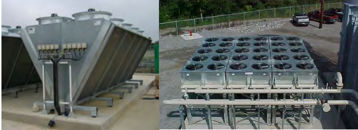
Figure 2-7. Examples of Closed-Loop Dry-Air Coolers
