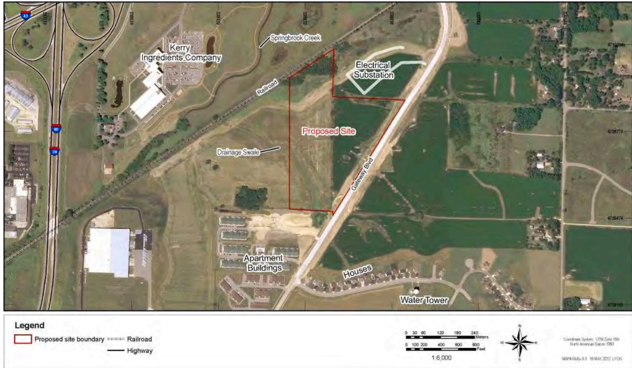
Figure 3-3. Aerial View of Visible Features Surrounding the Project Site
